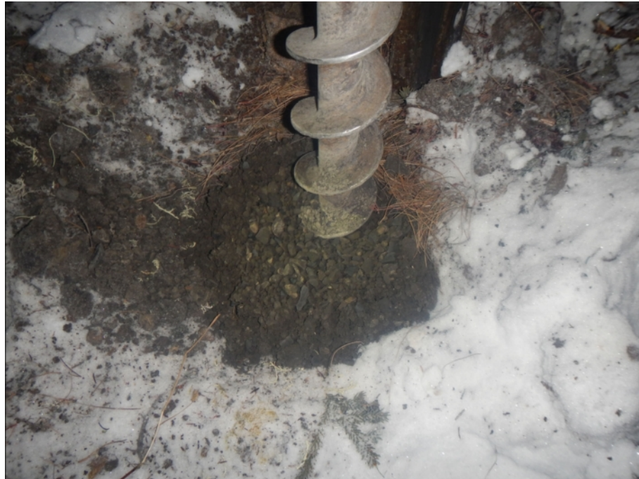
Figure 905-6597.1 Photo of drill cuttings coming up auger in borehole 904-6597 from 2.0 and 3.0m
