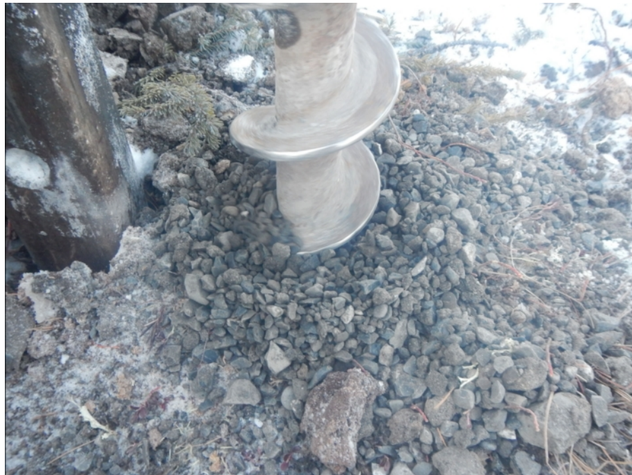
Figure 905-6601.2 Photo of auger cuttings coming up borehole 905-6601 from between 3 and 4.5m
