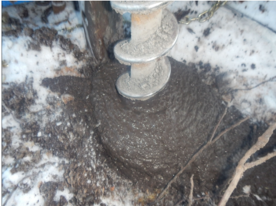
Figure 905-6596.1 Photo of drill cuttings coming up auger in borehole 904-6596 from 0 and 0.4m
