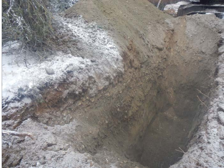
Figure 906-6573.1 Photo of test pit 906-6573
