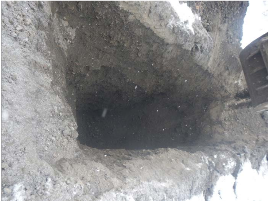
Figure 906-6568.2 Photo of test pit 906-6568
