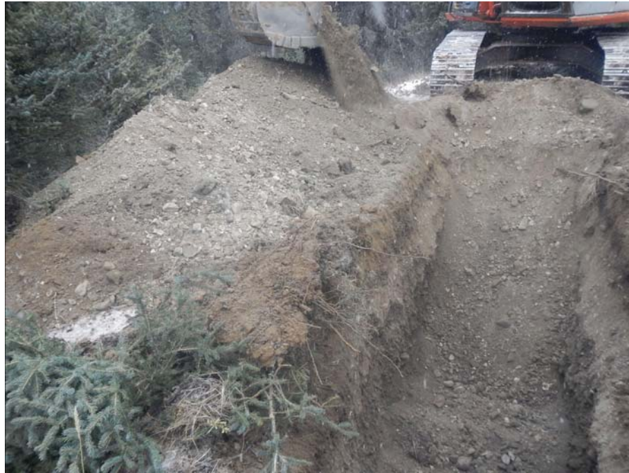
Figure 906-6562.1 Photo of test pit 906-6562
