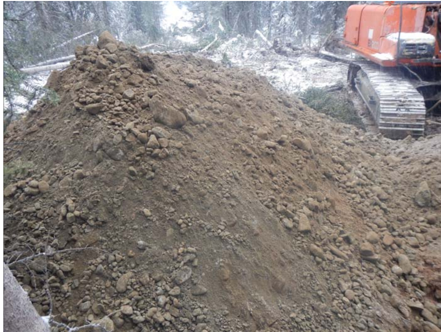
Figure 906-6571.1 Photo of waste pile from test pit 906-6571
