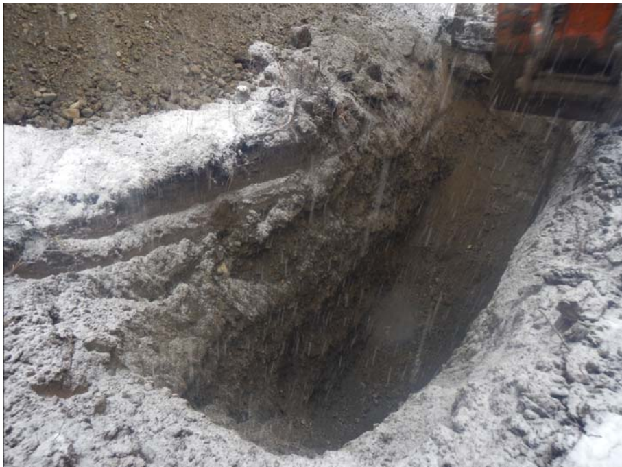
Figure 906-6567.2 Photo of test pit 906-6567
