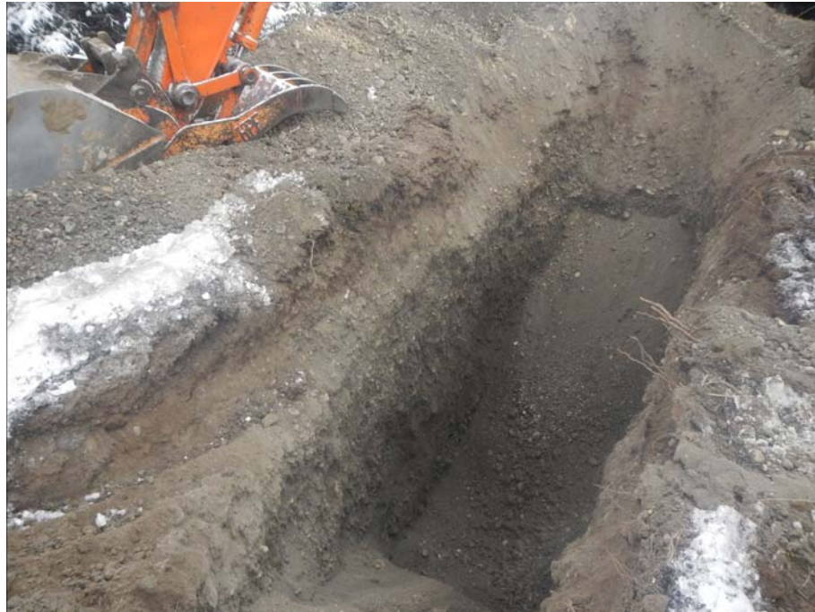
Figure 906-6572.1 Photo of test pit 906-6572
