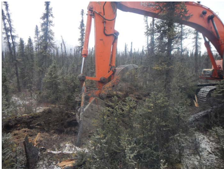
Figure 908-6555.2 Photo of excavation from test pit 908-6555
