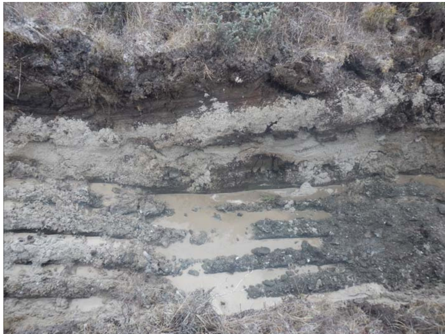
Figure 908-6553.2 Photo of test pit 908-6553
