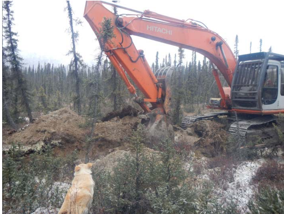
Figure 908-6558.1 Photo of excavation from test pit 908-6558
