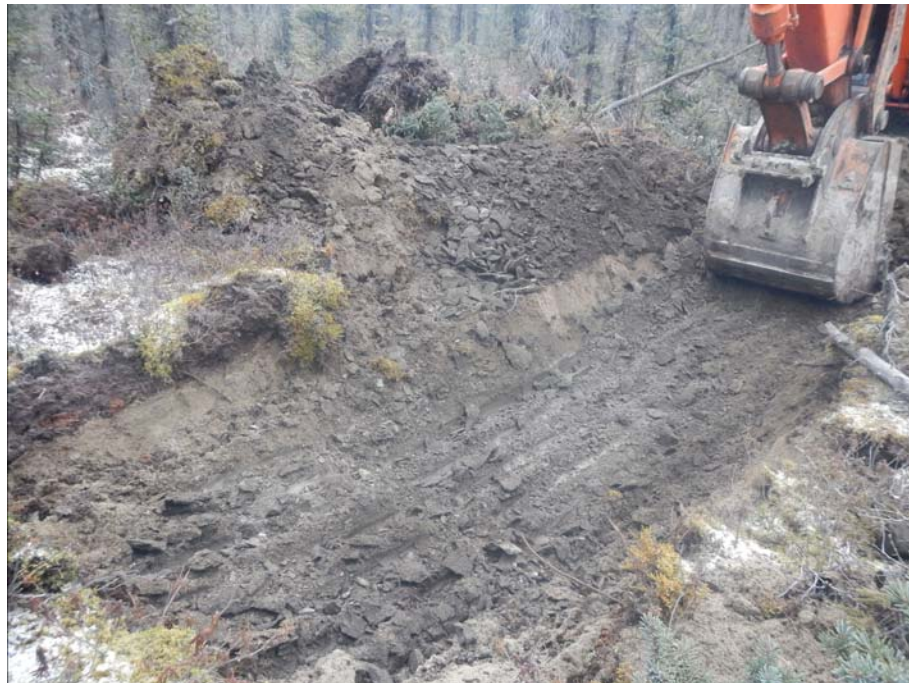
Figure 908-6556.2 Photo of test pit 908-6556
