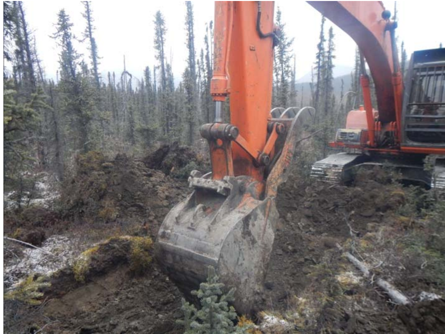
Figure 908-6556.1 Photo of excavation from test pit 908-6556
