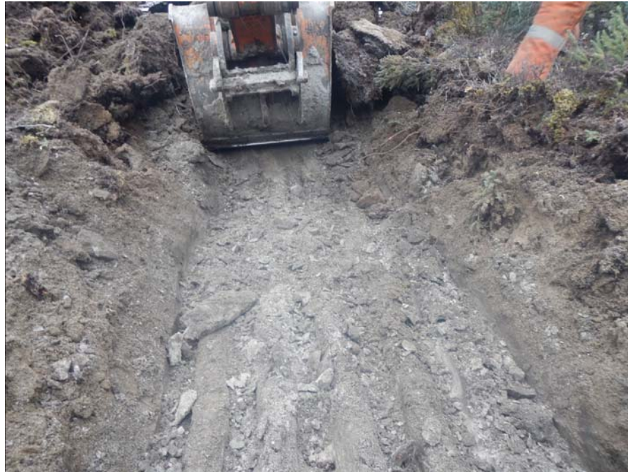
Figure 908-6554.1 Photo of test pit 908-6554
