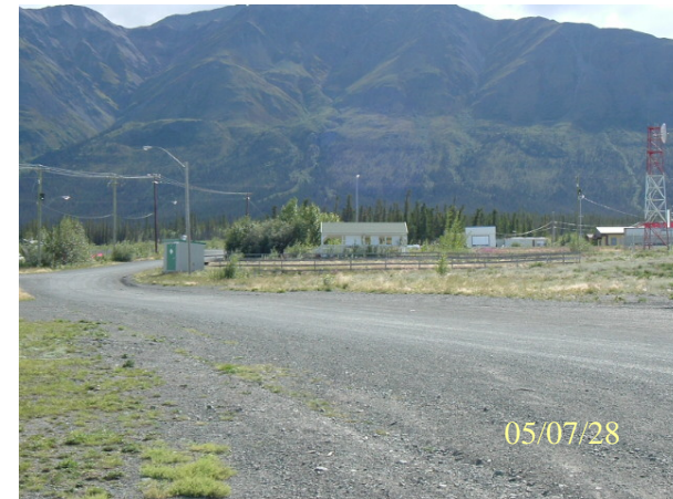
Photo 0590: 3957 Destruction Bay community septic system # 2
