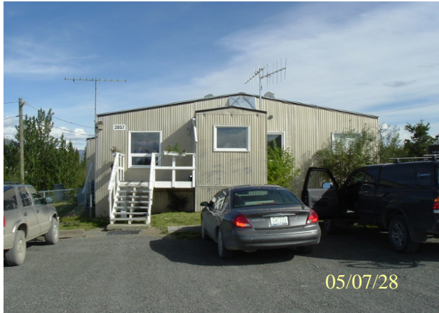
Photo 0586: 3957 Destruction Bay Health Centre
