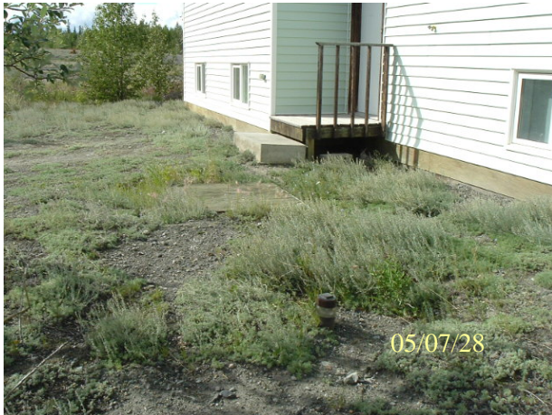
Photo 0597: 3957 Abandoned well nursing residence # 2 (back)
