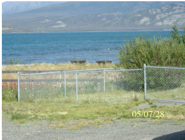
Photo 0588: 3957 Destruction Bay community septic system # 1
