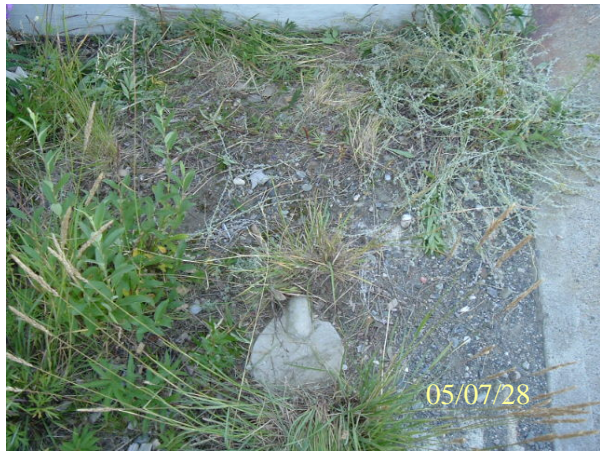
Photo 0584: 3201 Abandoned well adjacent to existing well
