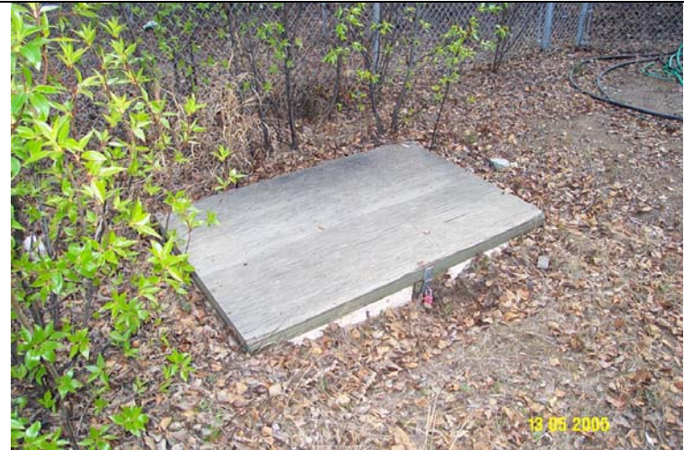
Photo 0158: 6511-C Irrigation Well Wellhead
