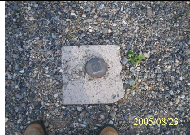
Photo 214: 5672 Potential septic clean out?
