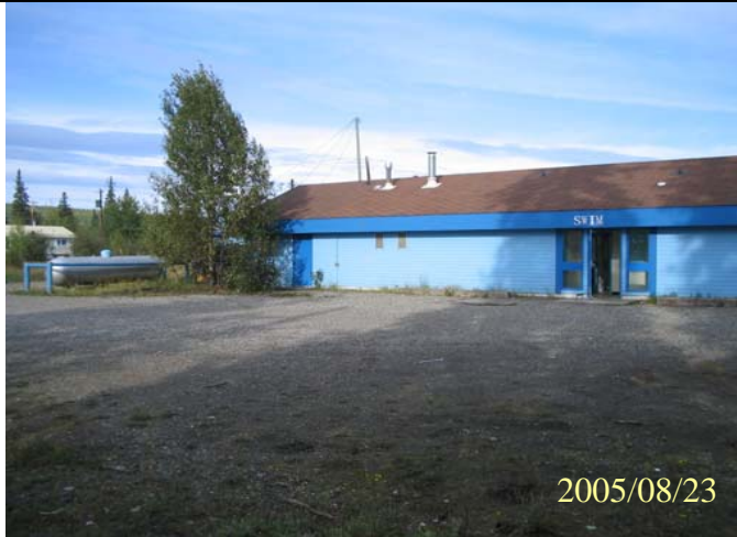
Photo 208: 5672 Pelly Crossing swimming pool. (northeast)
