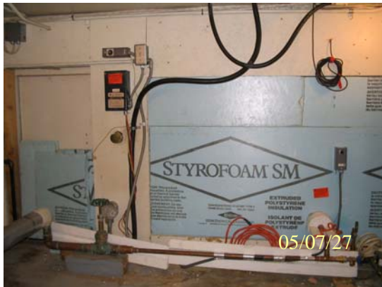
Photo 0083: 3122 Point of entry to Community Club
