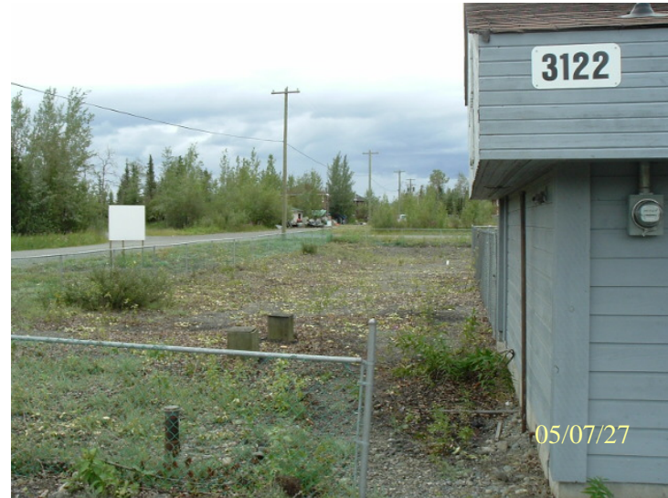
Photo 0542: 3122 Swimming pool septic field
