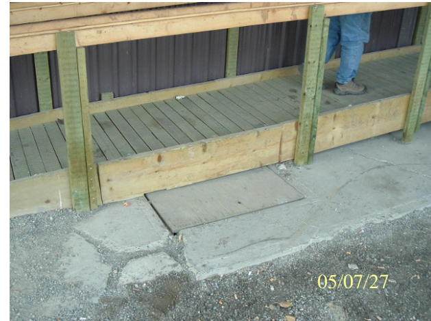
Photo 0537: 3122 Wellhead enclosure under wheelchair ramp
