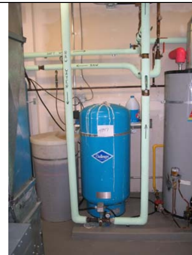
Photo 0028: 4951 Pressure tank
