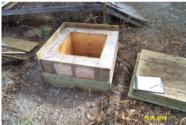
Photo 0192: 1955 Well Head Enclosure
