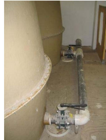
Photo 0022: 1955 Storage Tank Piping
