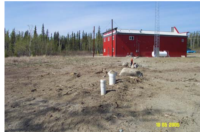
Photo 0094: 1421 Septic Field (front) and Mendenhall Firehall (back)
