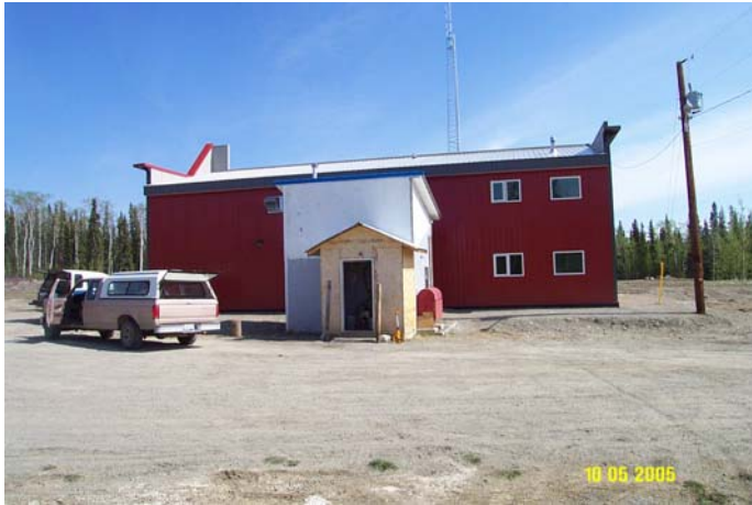
Photo 0091: 1421 Well house, Above Ground Storage Tank and Water-Pickup (front) and Mendenhall Firehall (back)
