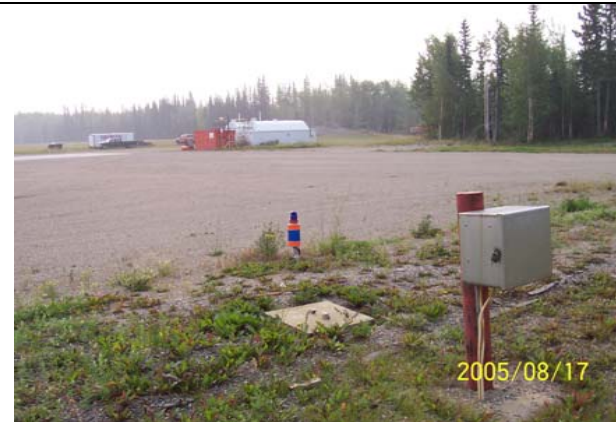
Photo 007: 5653 Septic tank (front) and bulk fuel storage (back).
