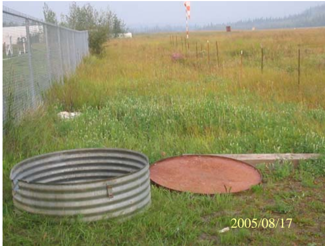
Photo 0187: 5653 Mayo Airport wellhead enclosure.
