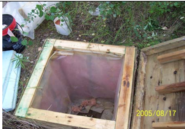
Photo 056: 5650 Wellhead enclosure.
