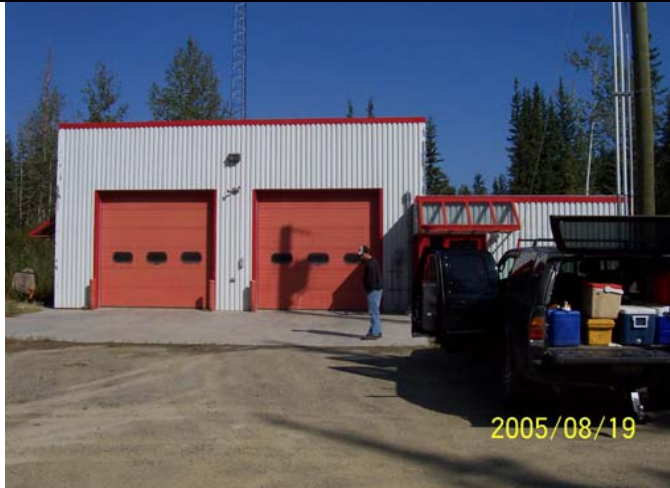
Photo 093: 2592 Klondike Valley Fire Hall
