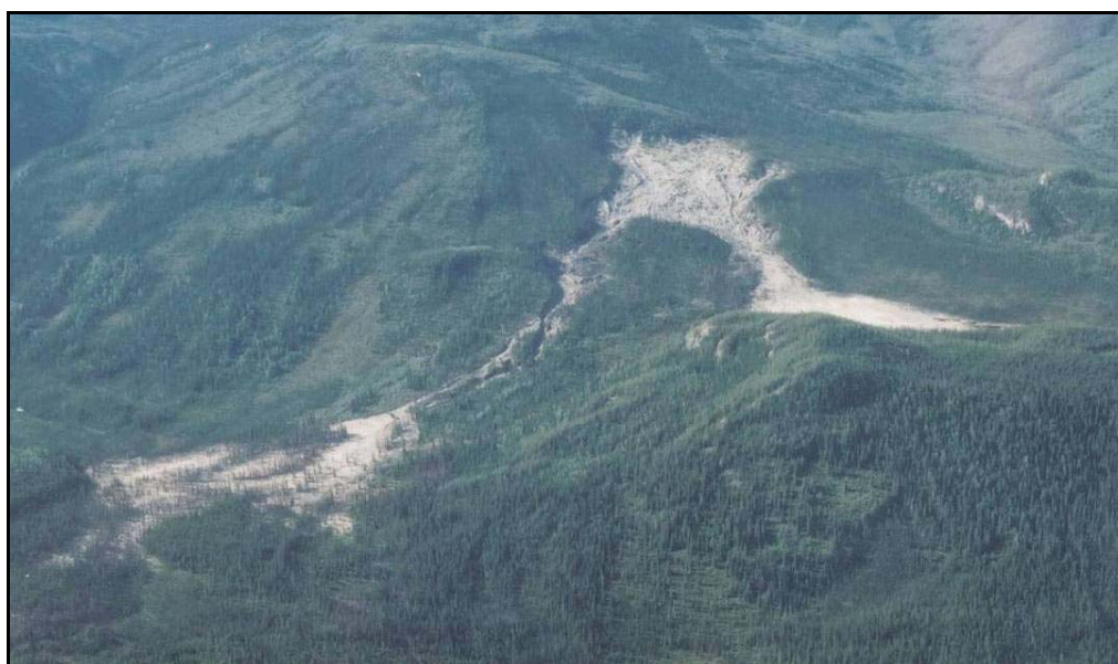
Figure 14 The Magundy Slide retrogressive thaw failure is comprised of three main components: the squarish source zone at the top of the slide (350 m wide), the smaller west fan deposition zone at the mid-right of the photo, and the larger east fan deposition zone in the lower left of the photo.
