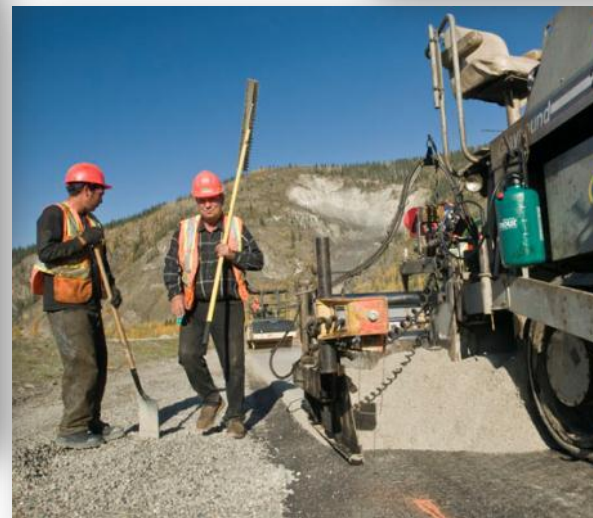
25 mm thick, top lift, pigmented asphalt
