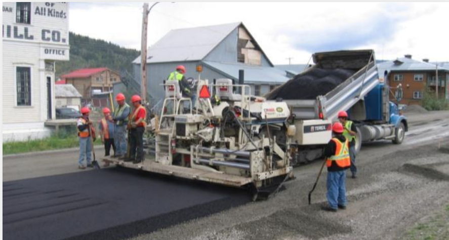
75 mm thick, bottom lift, standard black, asphalt cement
