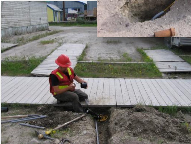
Thermistor Installation
