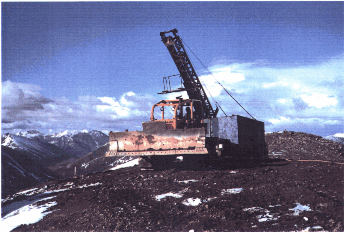
Diamond drill move - No.3 Zone
