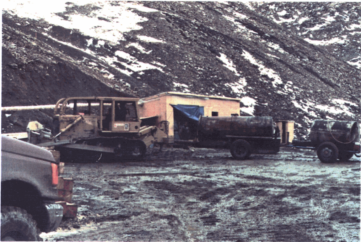
Cat train of fuel and water to portal
