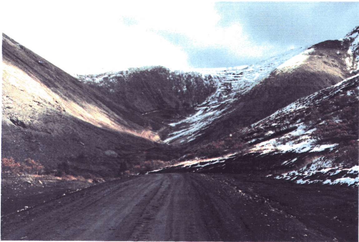
Portal access road (in distance) in early October, looking from Pass road north of camp
