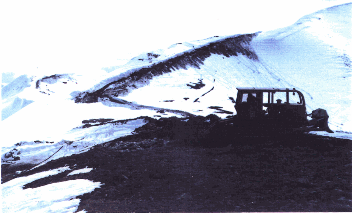
Diamond drill pad construction - Groundhog Zone
