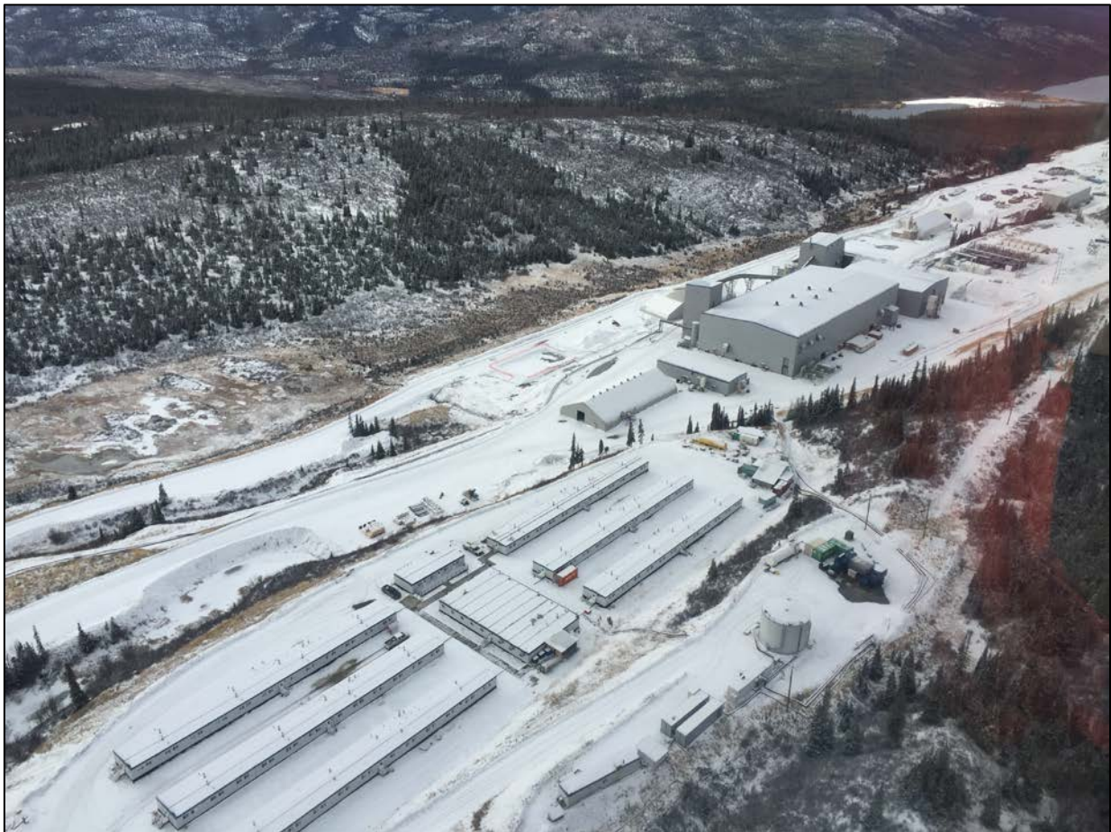
Figure 99: Overview of the Wolverine Mine and associated infrastructure
