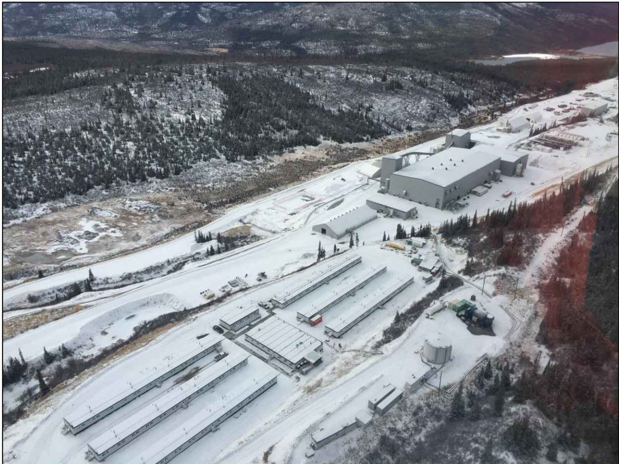
Figure 34: Overview of the Wolverine Mine and associated infrastructure
