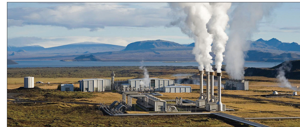
Geothermal power plant, Nesjavellir, Iceland.
