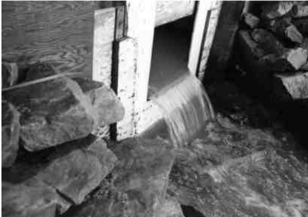
Figure 3.1. 0.3 m sharp-crested rectangular weir with end contractions installed at Galkeno 300 adit. Well-aerated, free falling nappe indicates suitability of weir to discharge volume.
