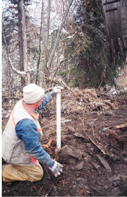
Plate 3: Typical Standpipe Piezometer Installation on Fence 3.
