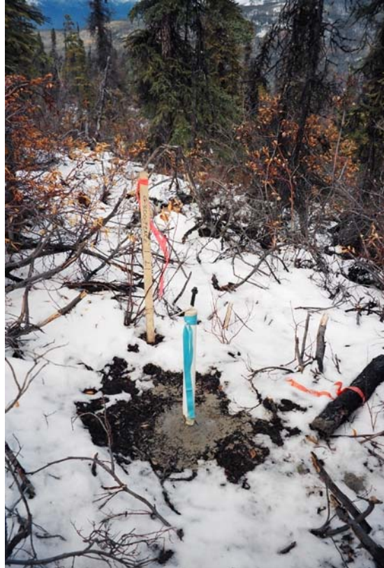
Plate 1: Typical Lysimeter Installation on Fence 1.
