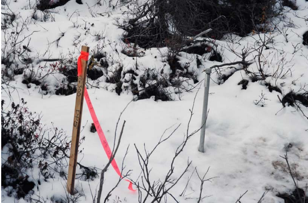
Plate 2: Typical Drive Point Piezometer Installation.
