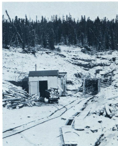
Adit driven into orebody for bulk sample for mill tests.
