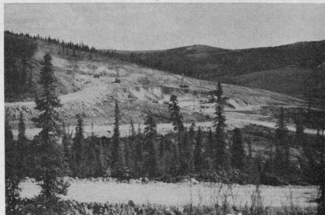
The first Anvil open pit; June, 1968.
