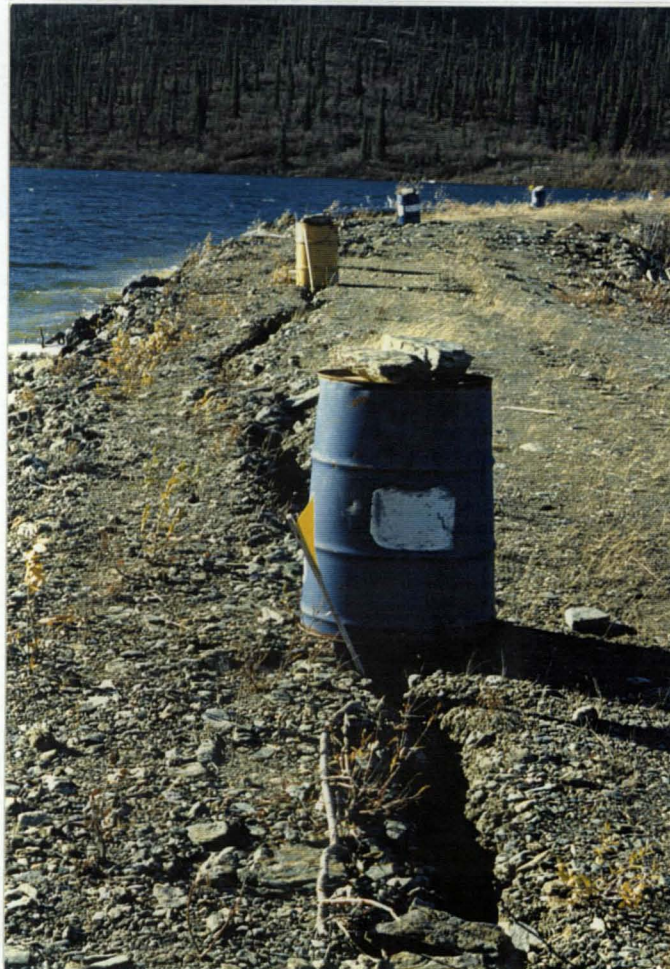
The upper photo illustrates the crest, looking south along the crest from near the spillway. The near-foreground blue barrel in this photo is captured by the lower photo, and the nature of the crest cracking can be noted.
