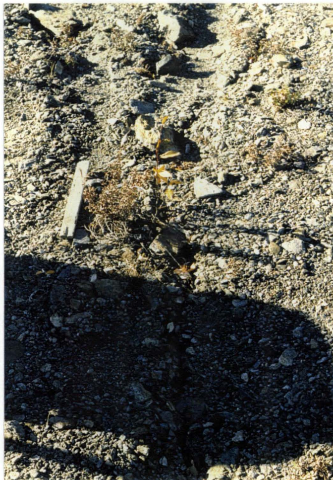
The upper photo shows a well-worn major crack at the edge of the crest, as well as 2 minor cracks farther to the right. The lower photo is a close-up of the test pit area immediately behind the barrel shadow. The lath can be used for scale to appreciate the width of the 1994/95 crack.
