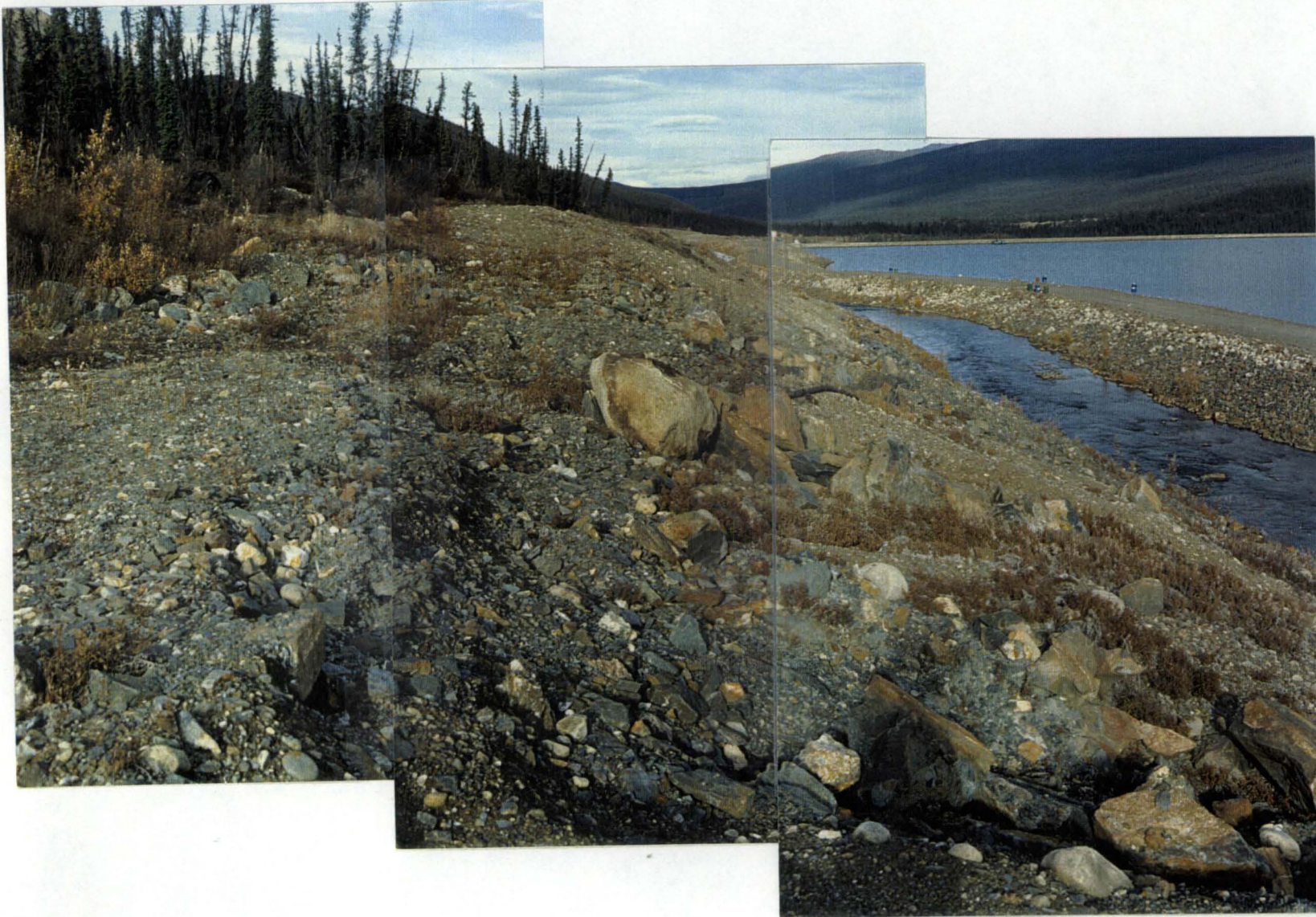
Looking downstream, the area in the central foreground has suffered displacement, beginning in 1991. It appears that there has been no movement during the past year. Note that a portion of the top of the thermal liner (to the left) is not involved in the movement. See next figure for further details.
