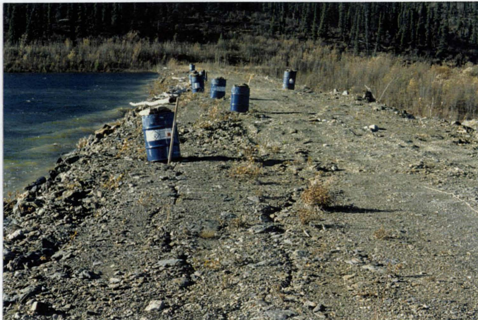
The upper photo shows a well-worn major crack at the edge of the crest, as well as 2 minor cracks farther to the right. The lower photo is a close-up of the test pit area immediately behind the barrel shadow. The lath can be used for scale to appreciate the width of the 1994/95 crack.
