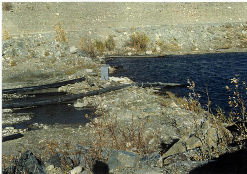
The upper photo illustrates the crest of the dam, looking northward. The lower photo is of the inlet to the spillway; the dyke may be retaining a pond level slightly above design FSL.
