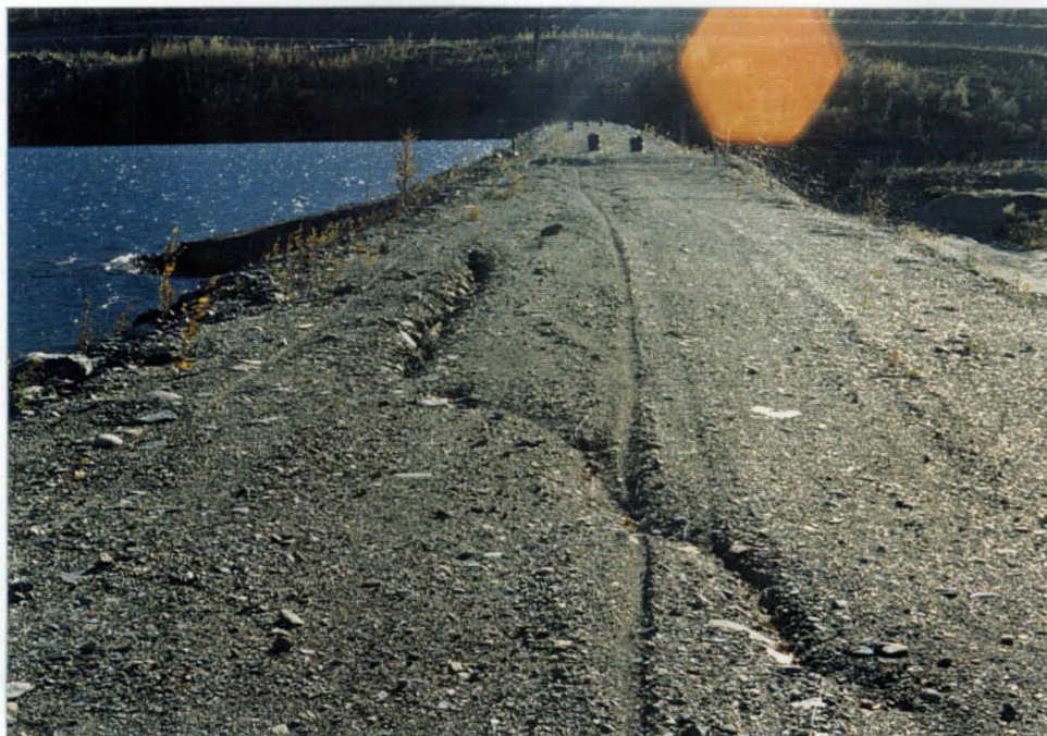
Looking southward along the crest, these photos illustrate the weathered status of old cracking. No sharp-edged cracks were observed.
