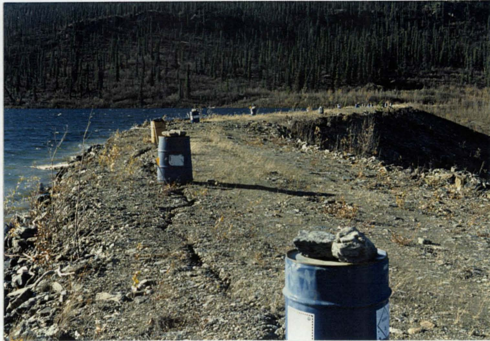
The upper photo illustrates the crest, looking south along the crest from near the spillway. The near-foreground blue barrel in this photo is captured by the lower photo, and the nature of the crest cracking can be noted.
