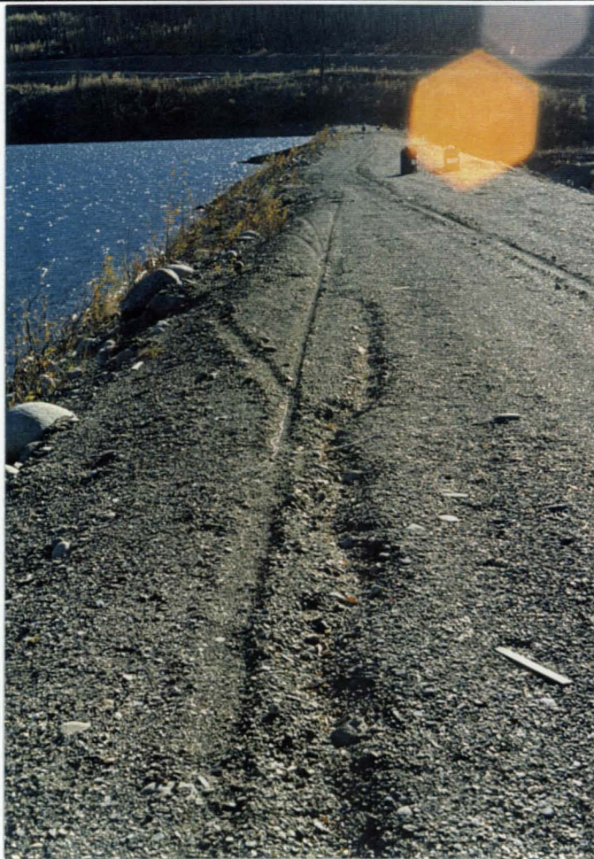
Looking southward along the crest, these photos illustrate the weathered status of old cracking. No sharp-edged cracks were observed.
