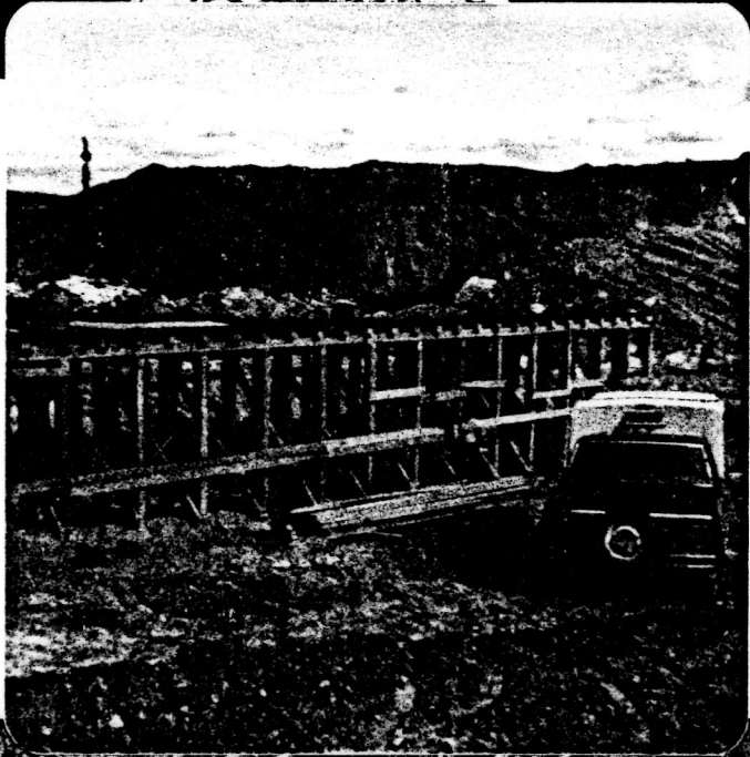
Dump Station Building Trestle
