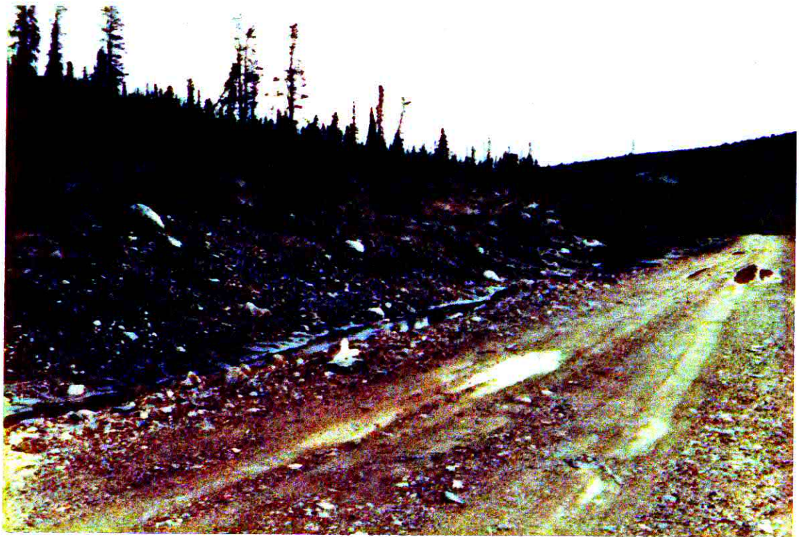
Photo 34 Groundwater seepage on west slope of Faro Creek Valley
