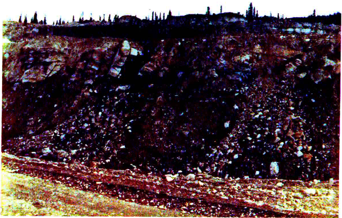
Photo 21 Transecting joints above overburden slump
