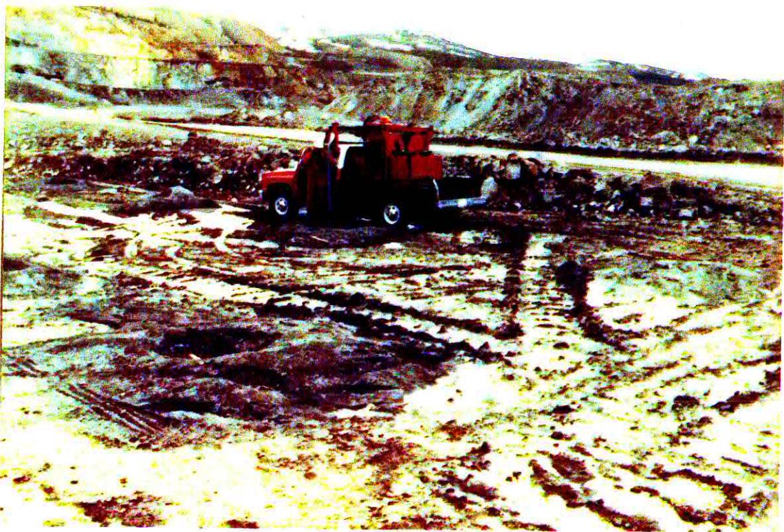
Photo 28 Pump test on 3870 bench
