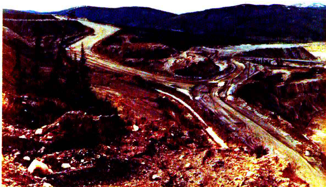
Photo 3 Lined ditches at edge of Zone 3 working area
