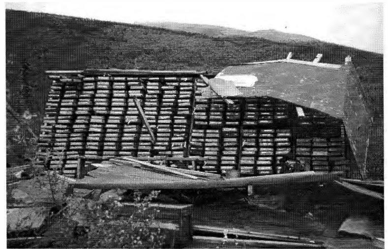
Plate 12. Collapsed core rack at the old Utah Mines' Maxi camp.
