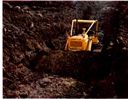
Illustration of a bulldozer trench being made across the 25 foot width of No. 3 Vein.
