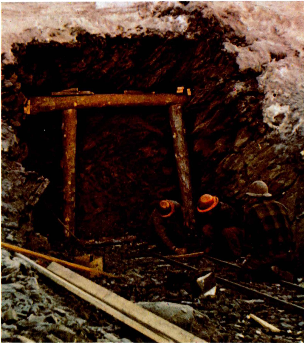
The first set at the portal site, preparatory to going underground.
