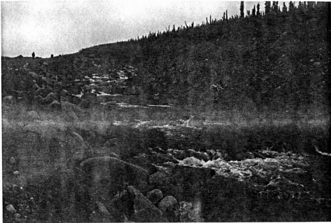
Photo 10: Upper segment of drop weirs. Note individual blocks displaced from their original positions.
