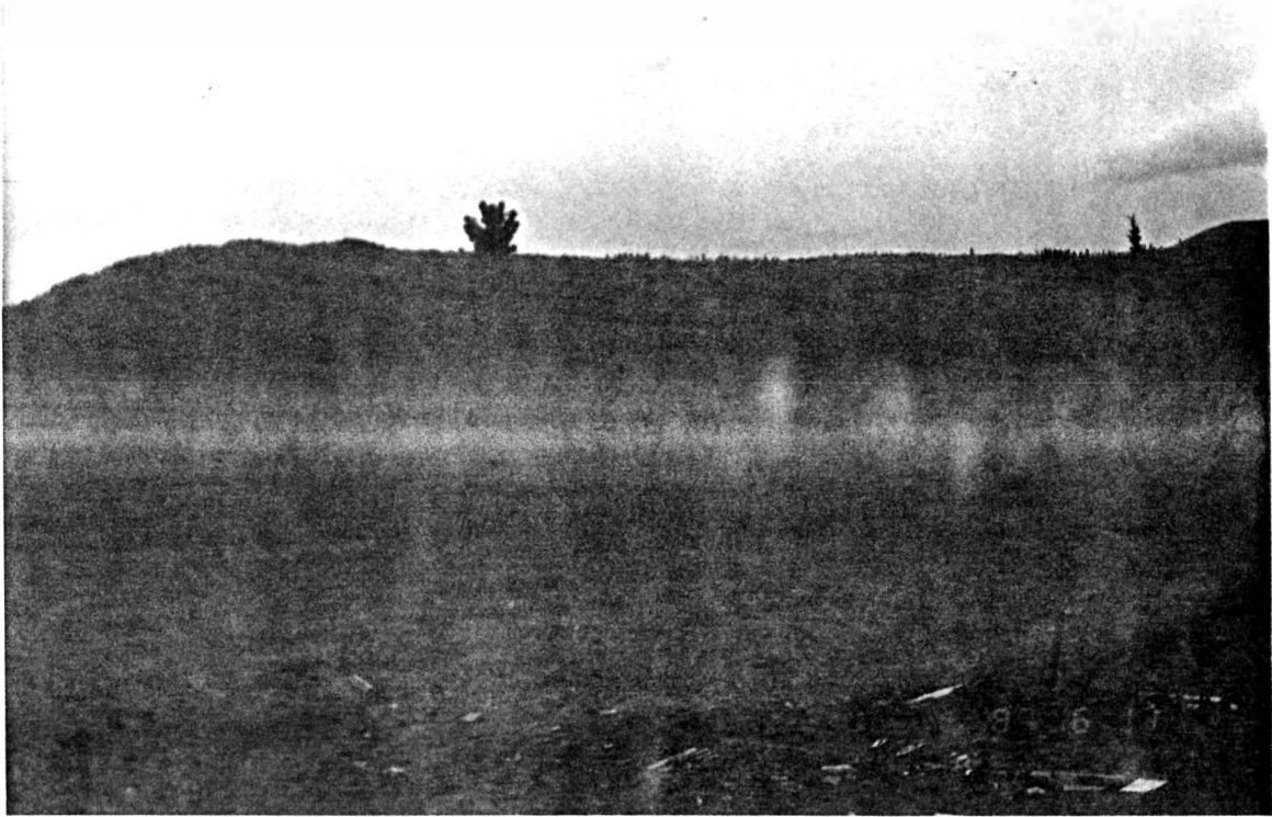
Photo 23: View of the proposed Grum Waste Dump area, looking across the Vangorda Creek valley.
