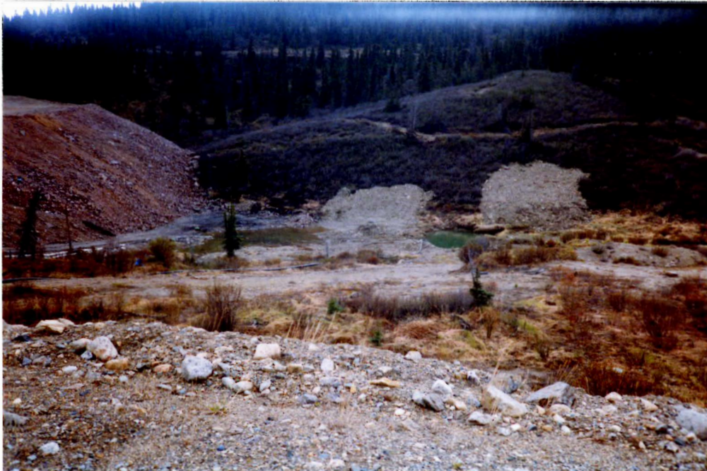
Photo 22 - North Fork seepage with excess zinc concentration ponded. I consider the upper waste pile slope can be covered with low permeability clay till and the valley be filled with waste rock.
