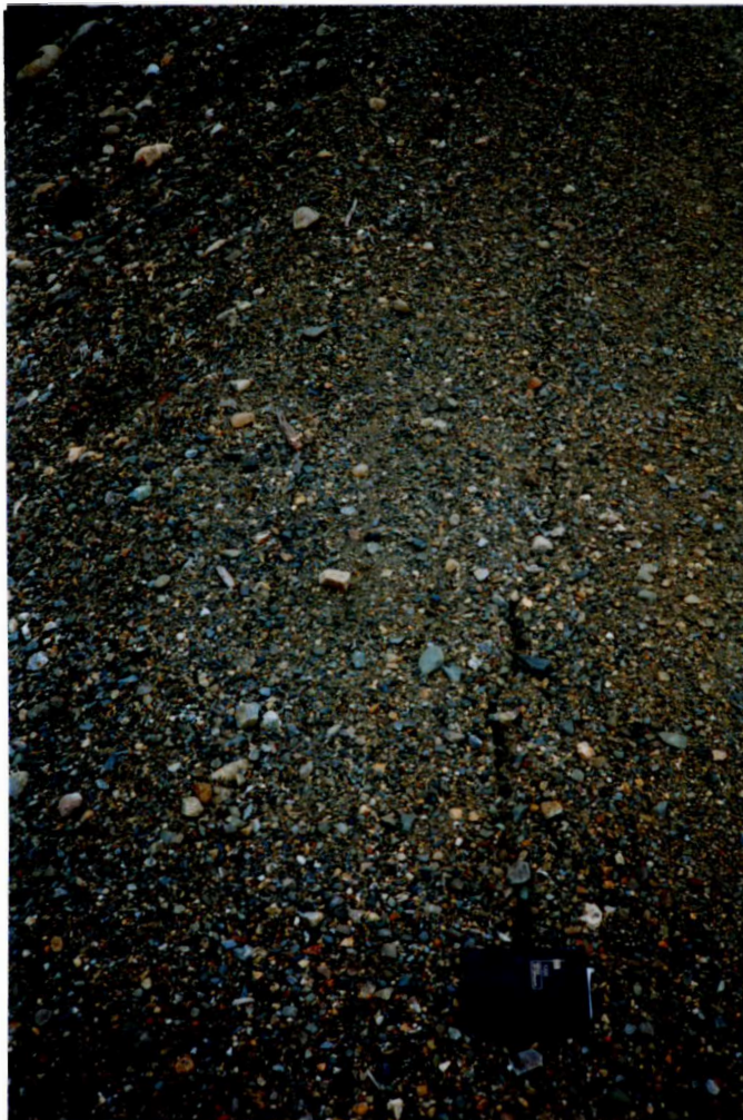
Photo 2 - Longitudinal crack on top of intermediate dam. Golder Associates consider these are due to frost heave. Note the water table is likely well below the surface. It is possible the dam foundation is spreading over thawed permafrost. The installation of movement monitors and thermistors is recommended.
