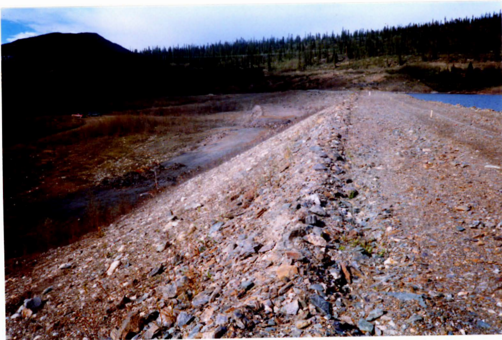
Photo 16 - Fresh water dam about 50 feet high.
