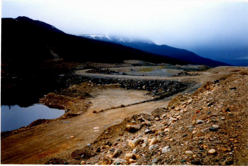
Photo 15 - Rose Creek diversion. The road elevation is lower than the dyke. It is recommended the several rip rap piles be positioned along the dyke in case emergency repairs are required quickly.
