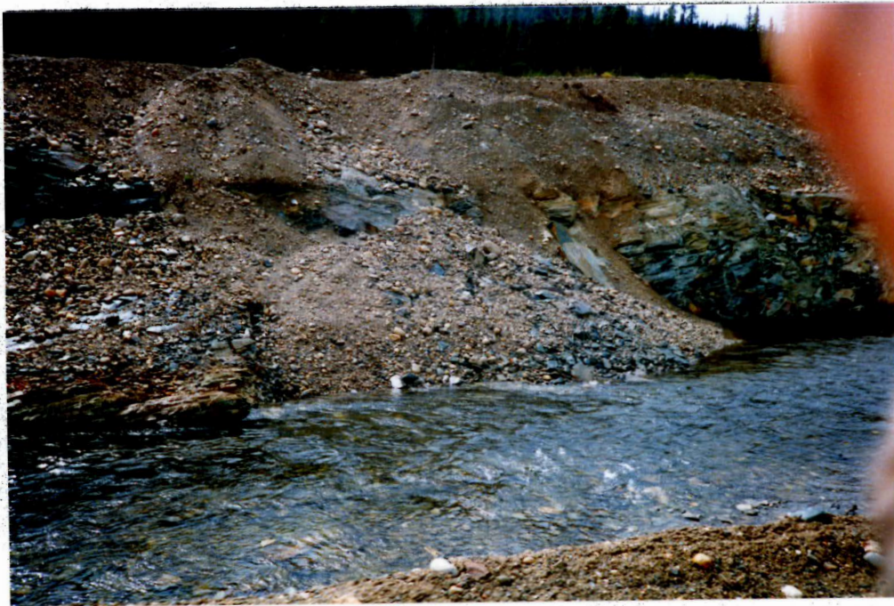
Photo 14 - Slope erosion partially filling in Rose Creek diversion. This material should be removed.
