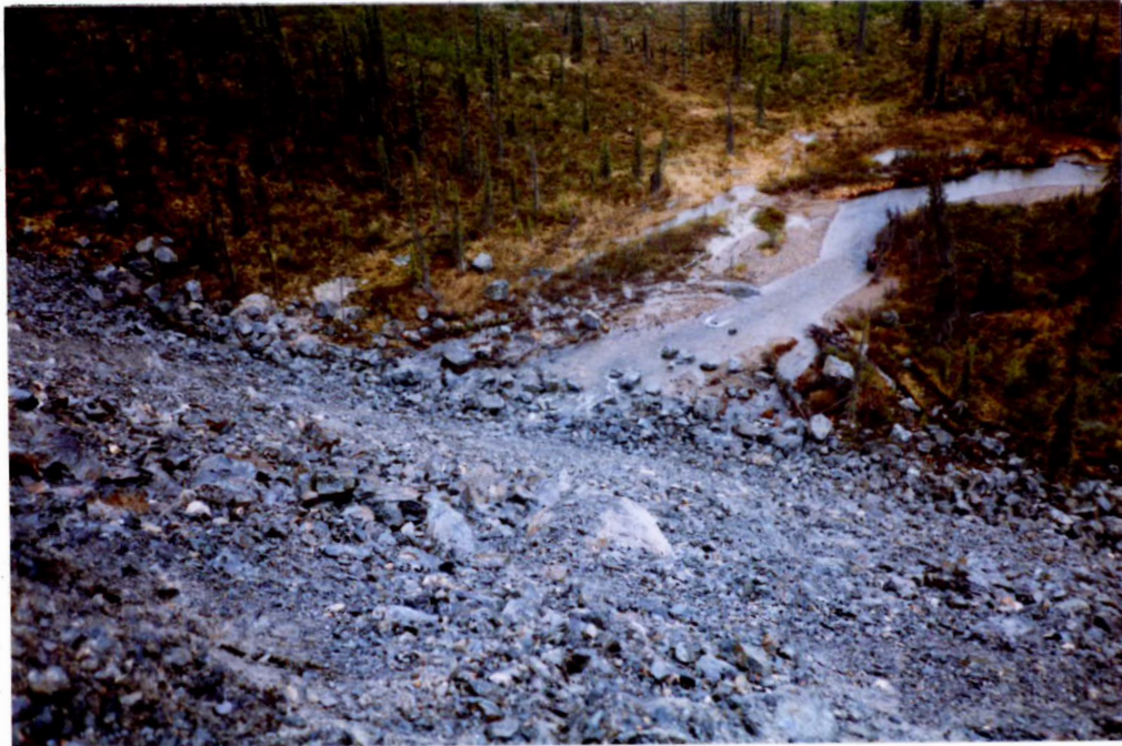
Photo 23 - North Fork flowing through a rock drain under the road being constructed to the Vangorda property. Properly constructed rock drains will operate effectively for short to moderate term. On abandonment the fill must be excavated and the creek channel redeveloped.
