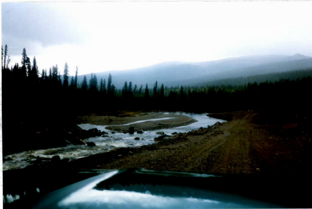
Photo 8 - The run out area of the Rose Creek diversion is developing scour and building a delta. This area should be stabilized.
