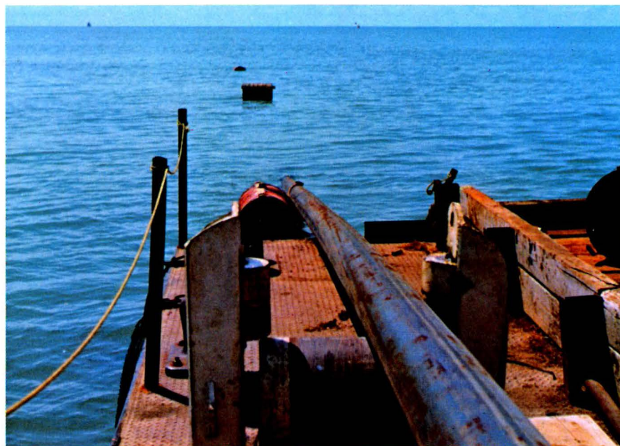
Laying pipeline in Lake Erie.
