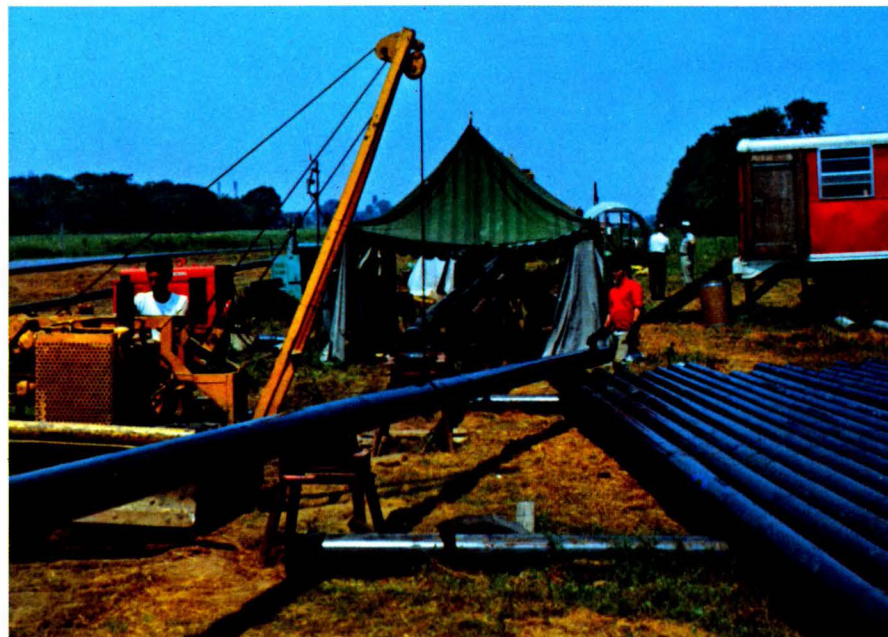
Assembling pipe on shore.
