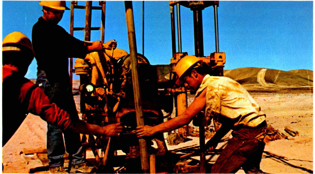
Diamond drilling at Sierra Gorda Project, February 1970.
