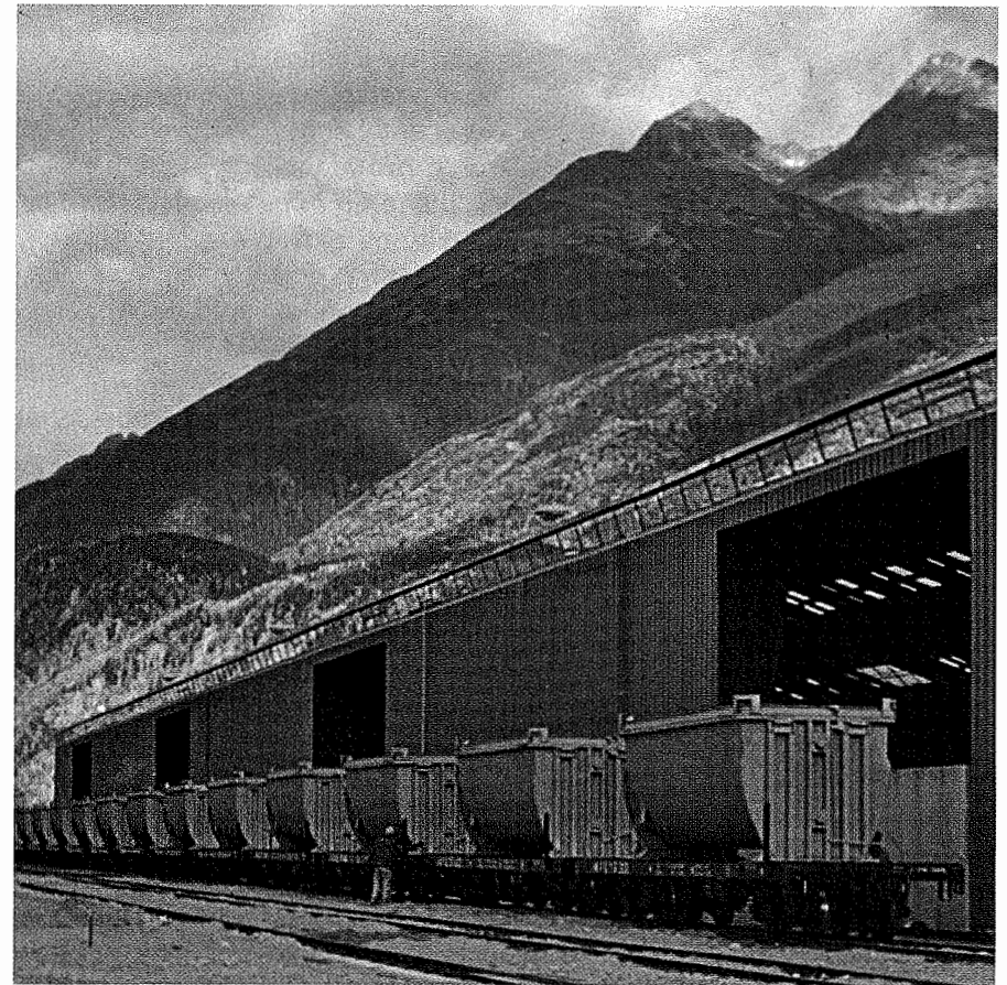
Containerized concentrates are shipped by truck and rail to port of Skagway.
