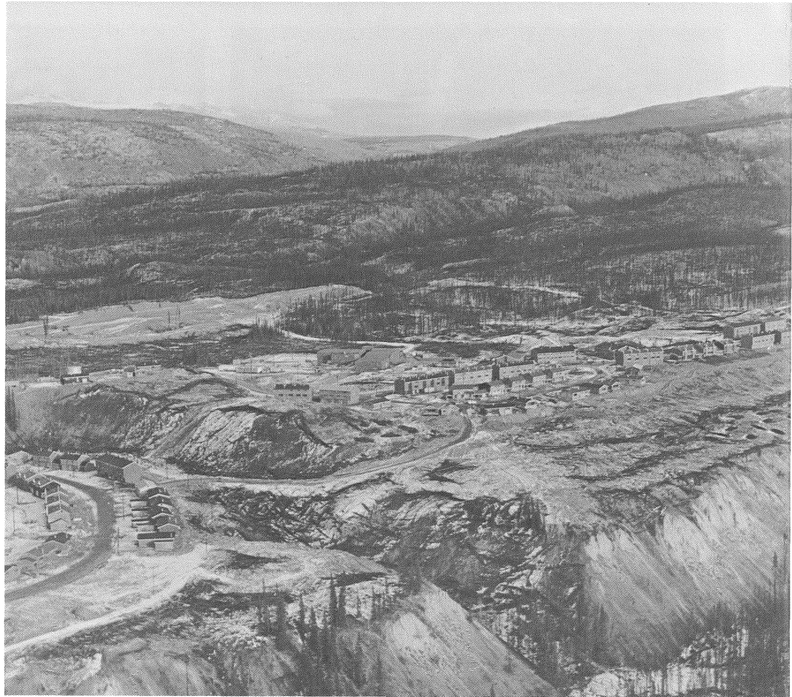
The new town of Faro carved out of the wilderness, a joint effort of Anvil and the Yukon Territorial Government.
