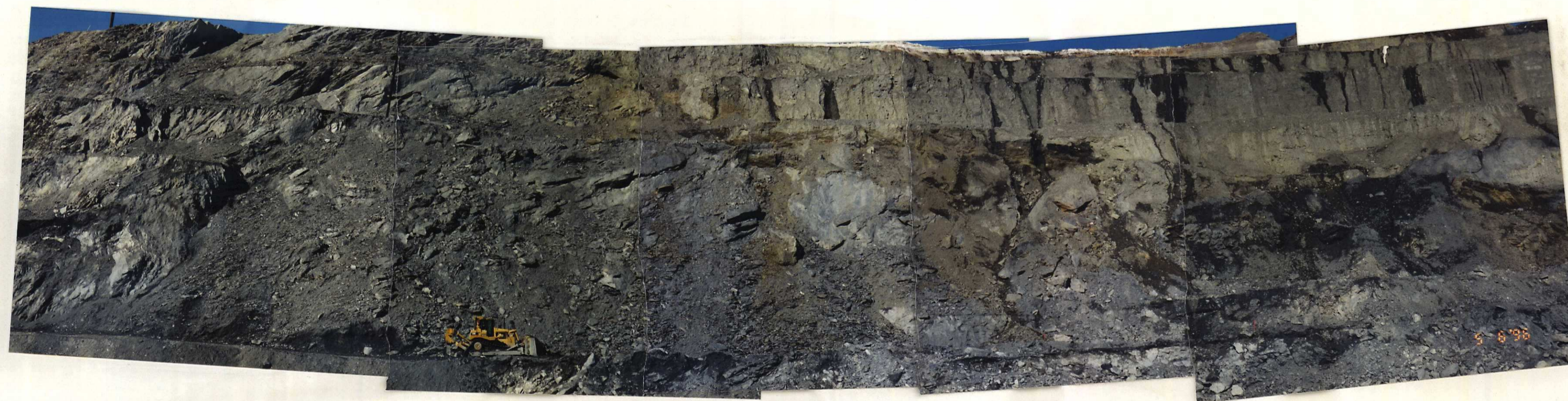
May 6, 1996: Dozer on 1216 Bench
