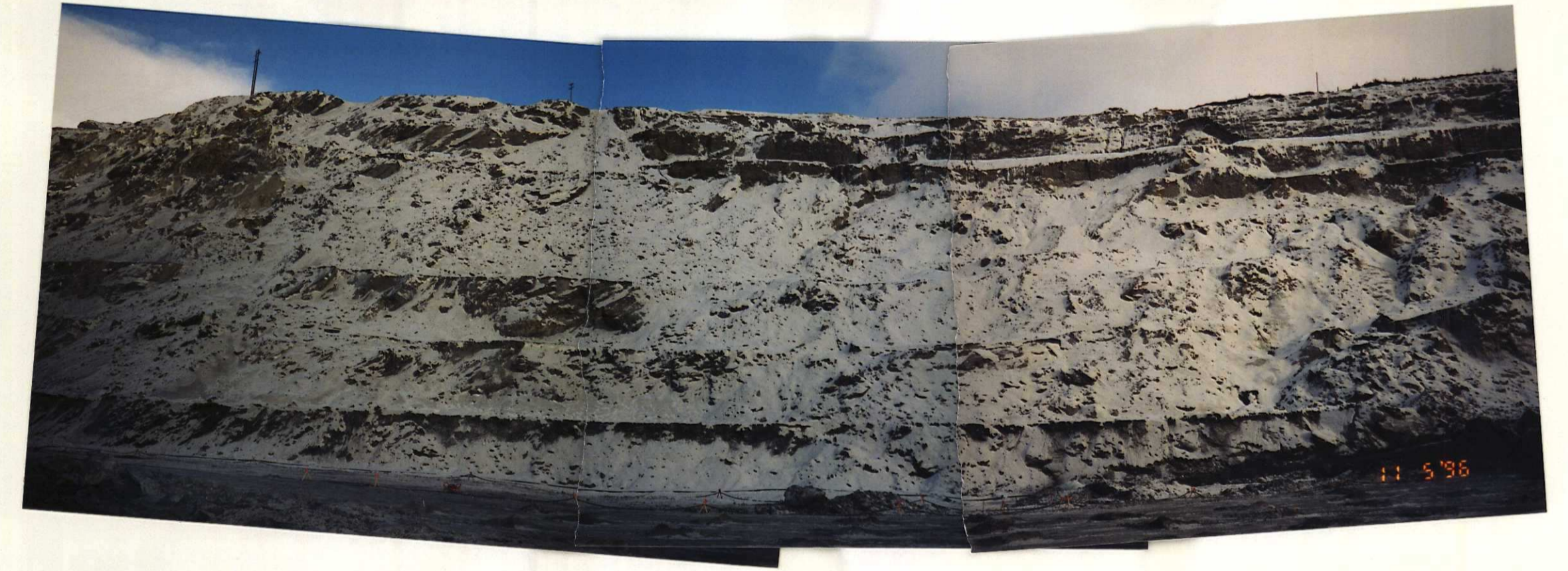
November 5, 1996: Power cable on 1186 Bench
