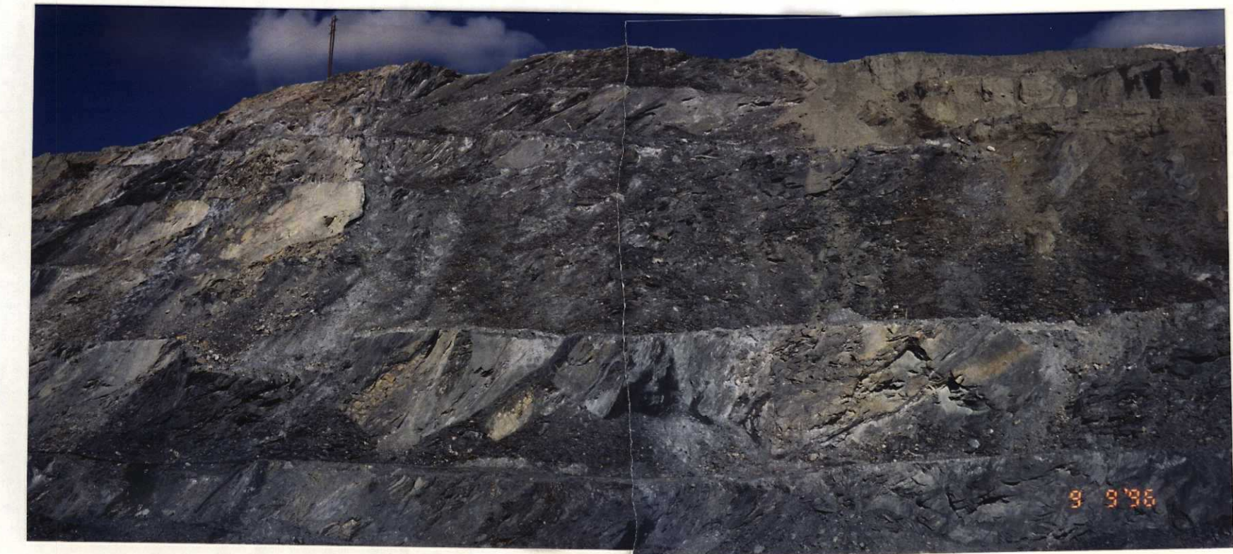
September 9, 1996: Pipe on 1204 Bench
