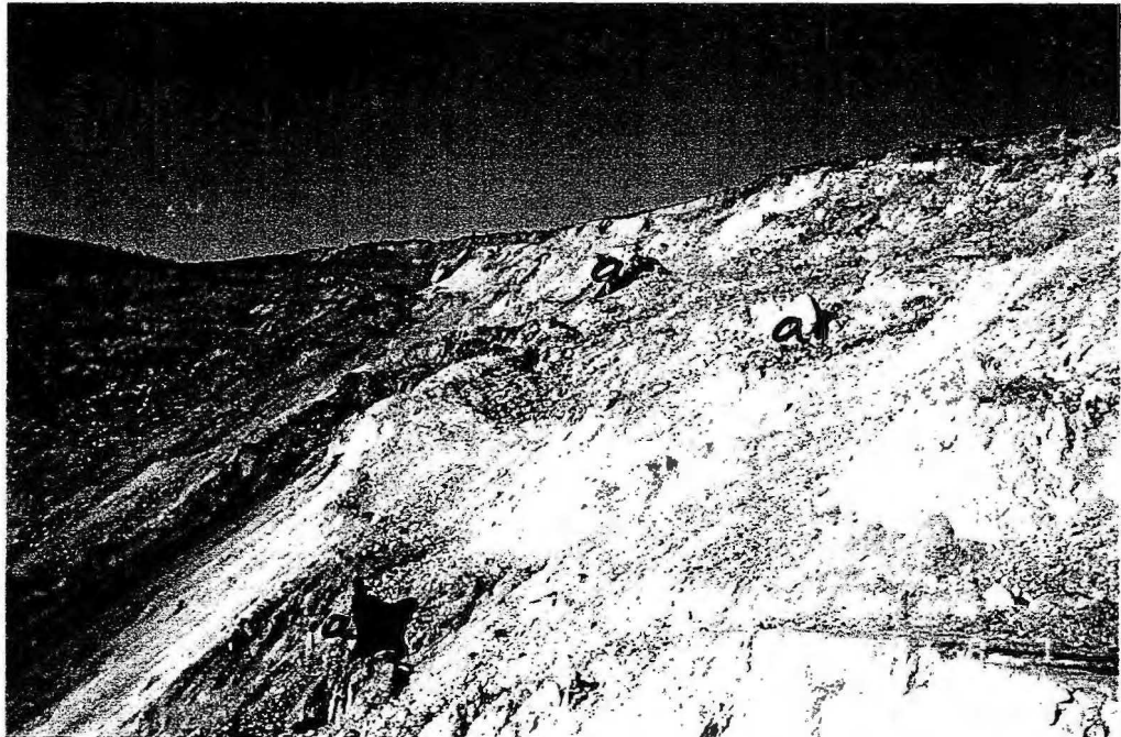
PHOTO 7: Side view of the upper slope. Note the protruding blocks which are evidence of toppling (a).
