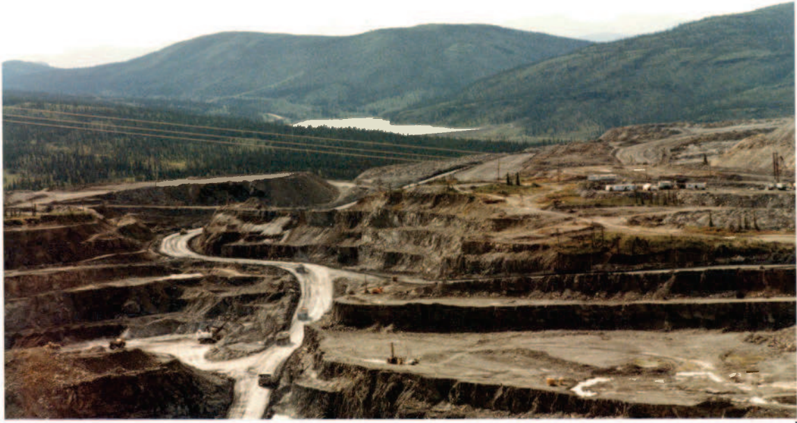
View from north wall of pit August 8/86 looking south, reservoir in background
