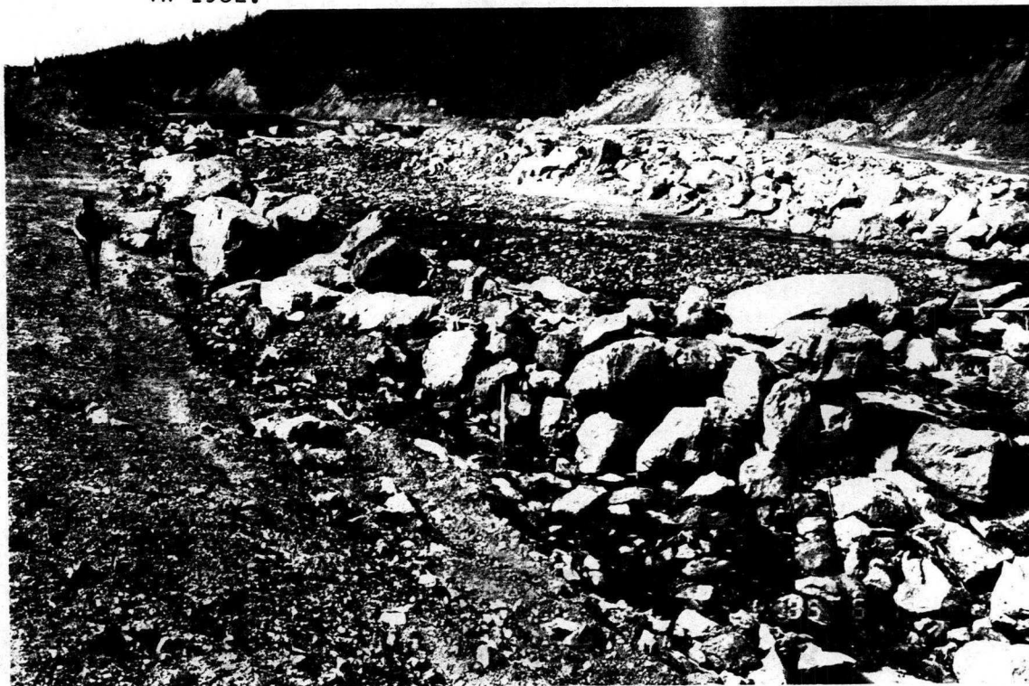
Photo 8: The rock-lined stream section (re-constructed in 1984) shows signs of erosion in 1986.
