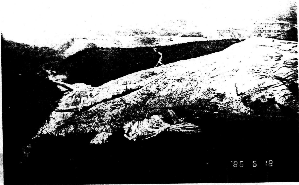
Photo 14: North lobe of the tailings pile reached the valley bottom and almost blocked the valley in June, 1986.
