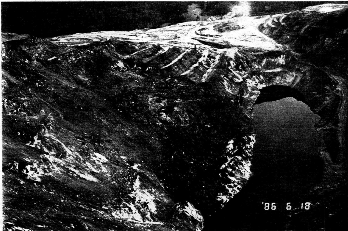
Photo 2: Porcupine Pit looking north. Note unstable west and south walls.
