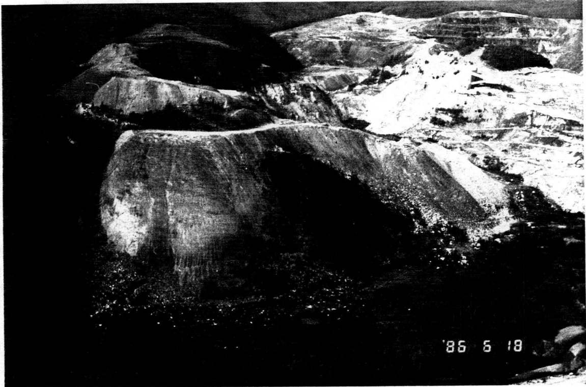
Photo 11: Snowshoe Pit waste dump deposited over the Clinton Creek valley. The dump is unstable - note the bulging.
