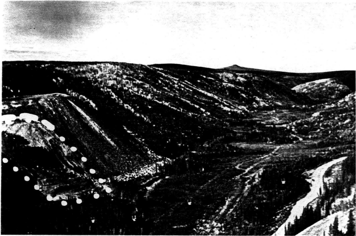
Photo 3: Clinton Creek and the waste dump, probably in 1970. Note slide on left side of the dump.
