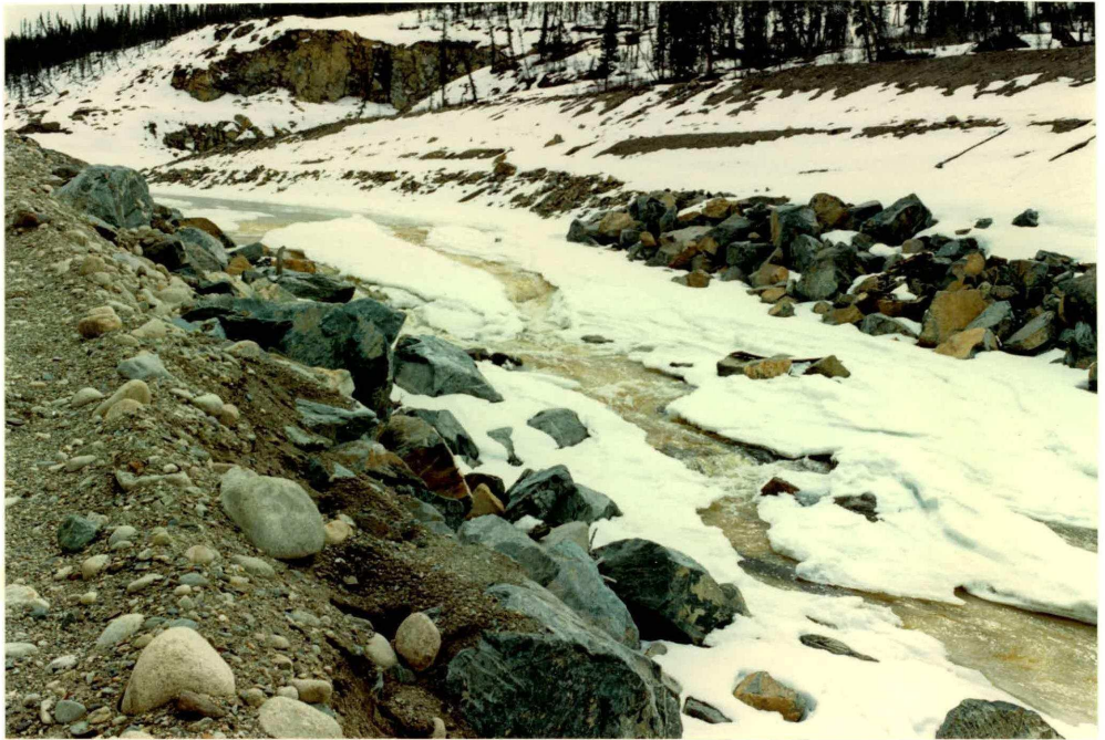
Plate 3. Upper Extent of Rose Creek Diversion Channel.
