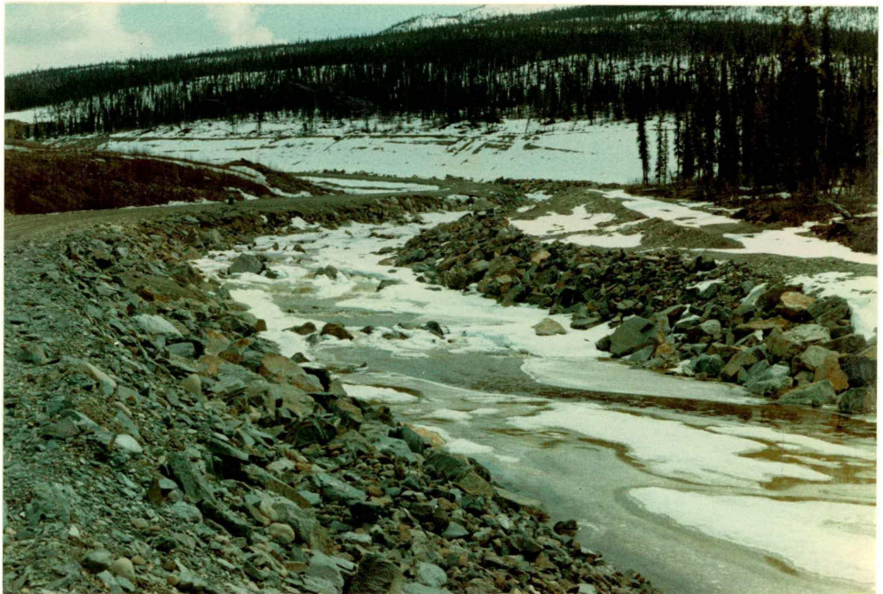
Plate 4. Mid-section of Rose Creek Diversion Channel.
