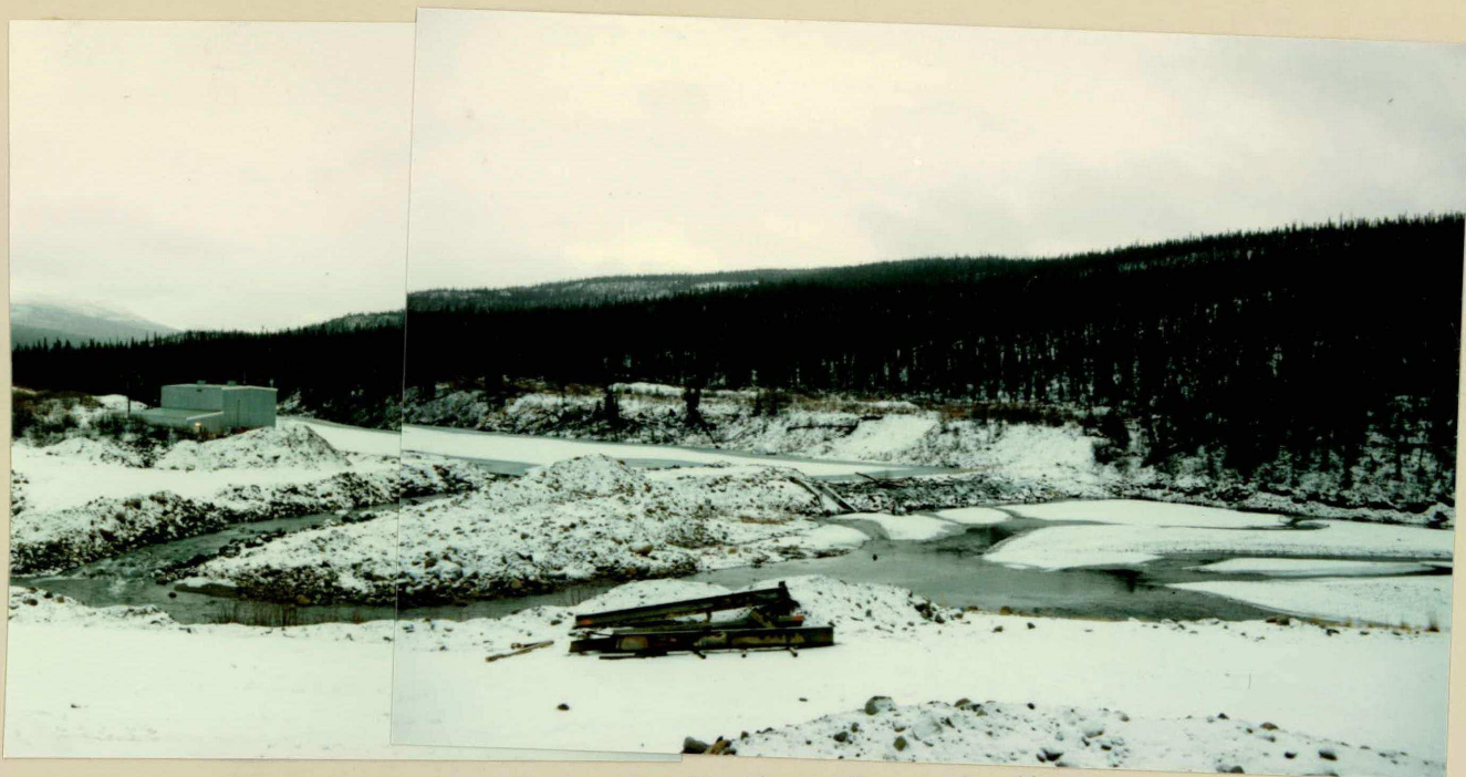
Photo One: Location of Station One at the Outflow of the Pumphouse Reservoir.
