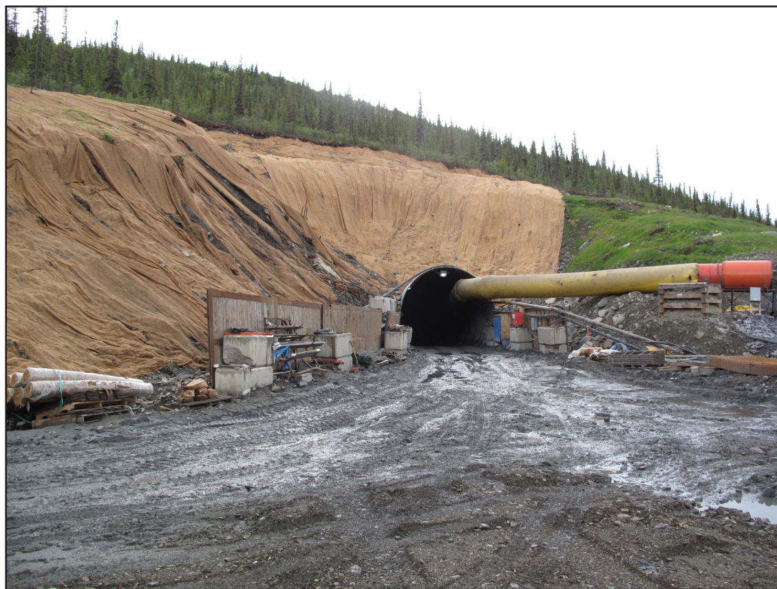
Bellekeno mine portal, Keno Hill silver property.
