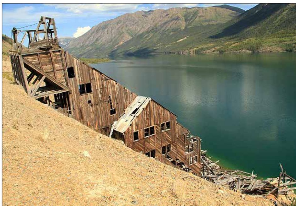
Historic mill and ore loading facilities of the Venus mine on the Windy Arm of Tagish Lake.
