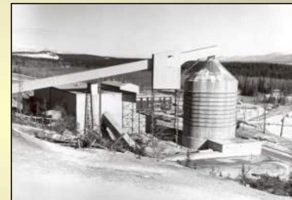
New Imperial Mines Ltd.: Surface buildings, circa 1970. The cylindrical tank was a storage bin for finely crushed ore.
