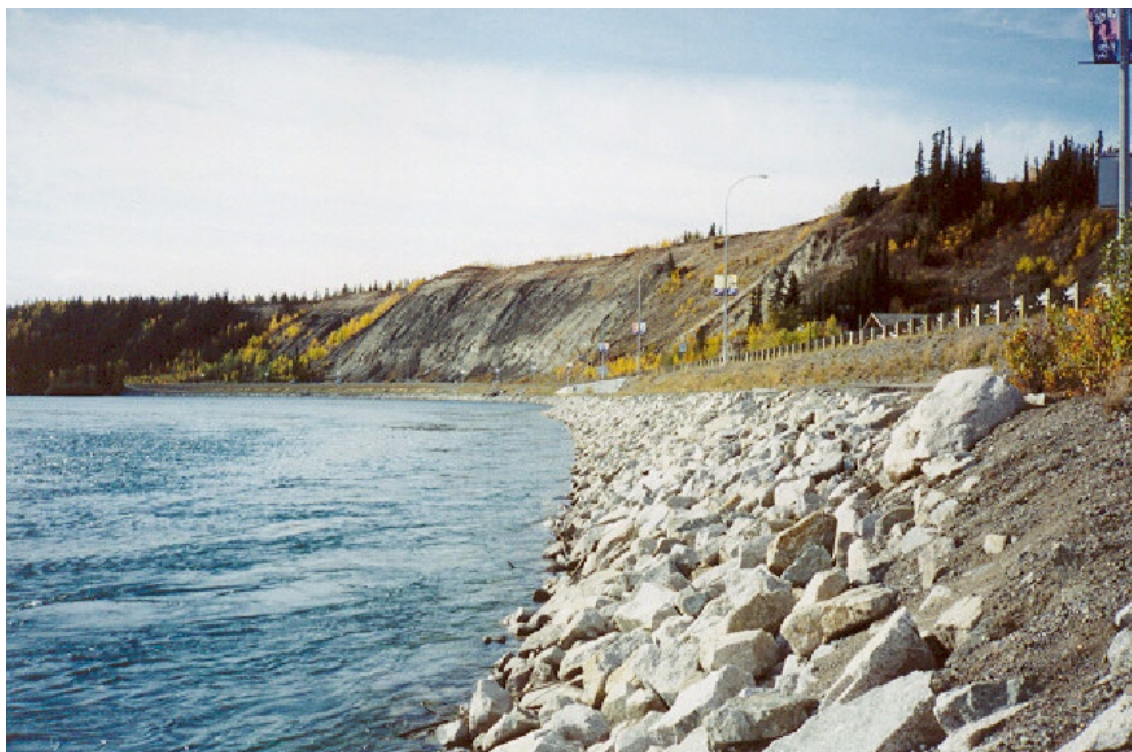
Plate 5. 'Granite' Rubble Used to Construct Breakwater along the Yukon River, Whitehorse, Yukon Pla5
