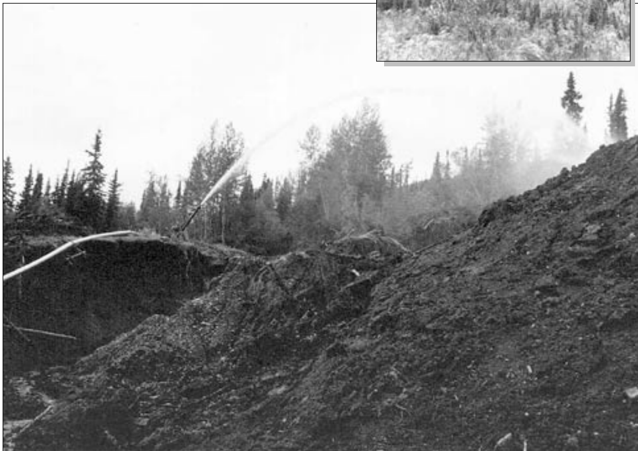
Bench during hydraulic stripping in 1986. (inset) Same area in August 1991, five years after revegetation.
