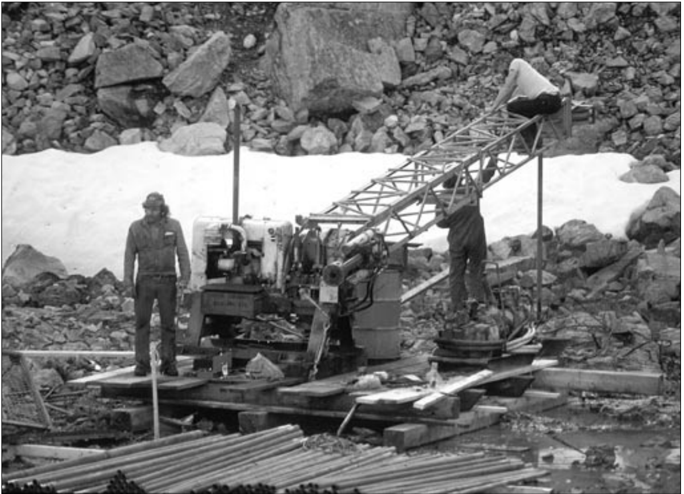
Working on a diamond drill.
