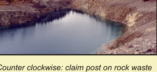
The linear shape of the mined-out pit shows that the deposit was a steep and narrow lens, roughly parallel to bedding. It now provides a popular summer swimming hole.
