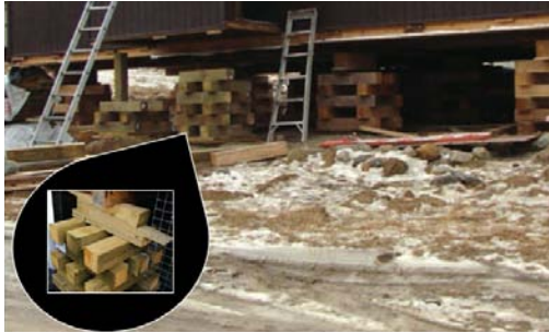
Figure F12. Example of a timber-block foundation used in Nunavut (Government of Nunavut, 2013).
