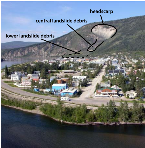
Figure 41 (above). The ‘Moosehide Slide’, or Dawson City Landslide, as seen from the Klondike River, showing the headscarp, central landslide debris, and lower landslide debris which has been modified by development.
