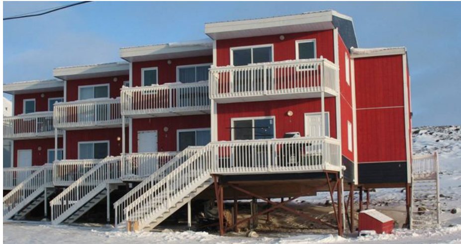
Figure F14. Example a steel-pile foundation in Nunavik (Gravel, 2012).
