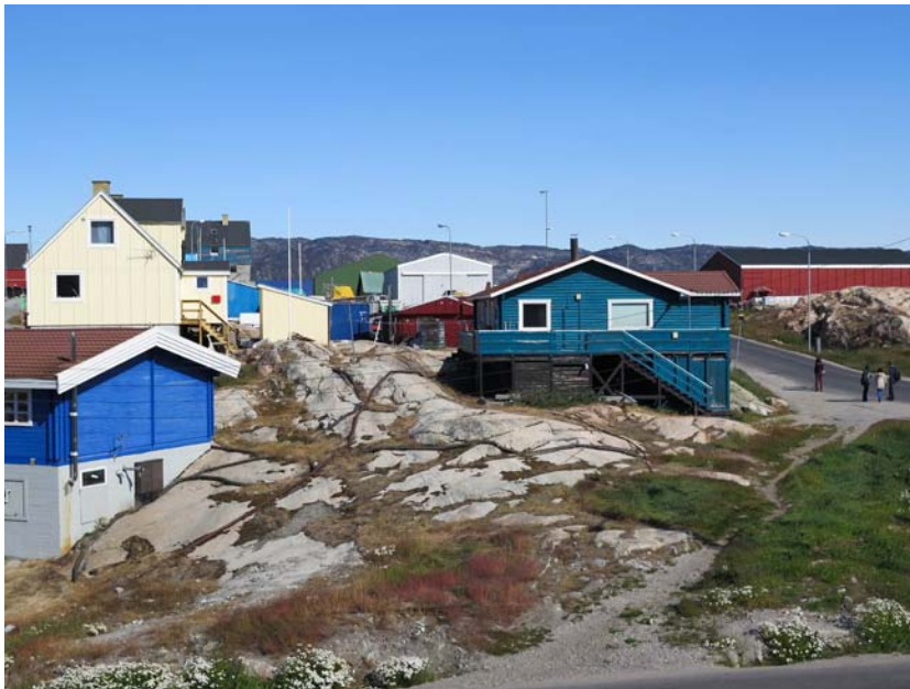
Figure F1. Houses in Ilulissat, western Greenland, built directly on bedrock.
