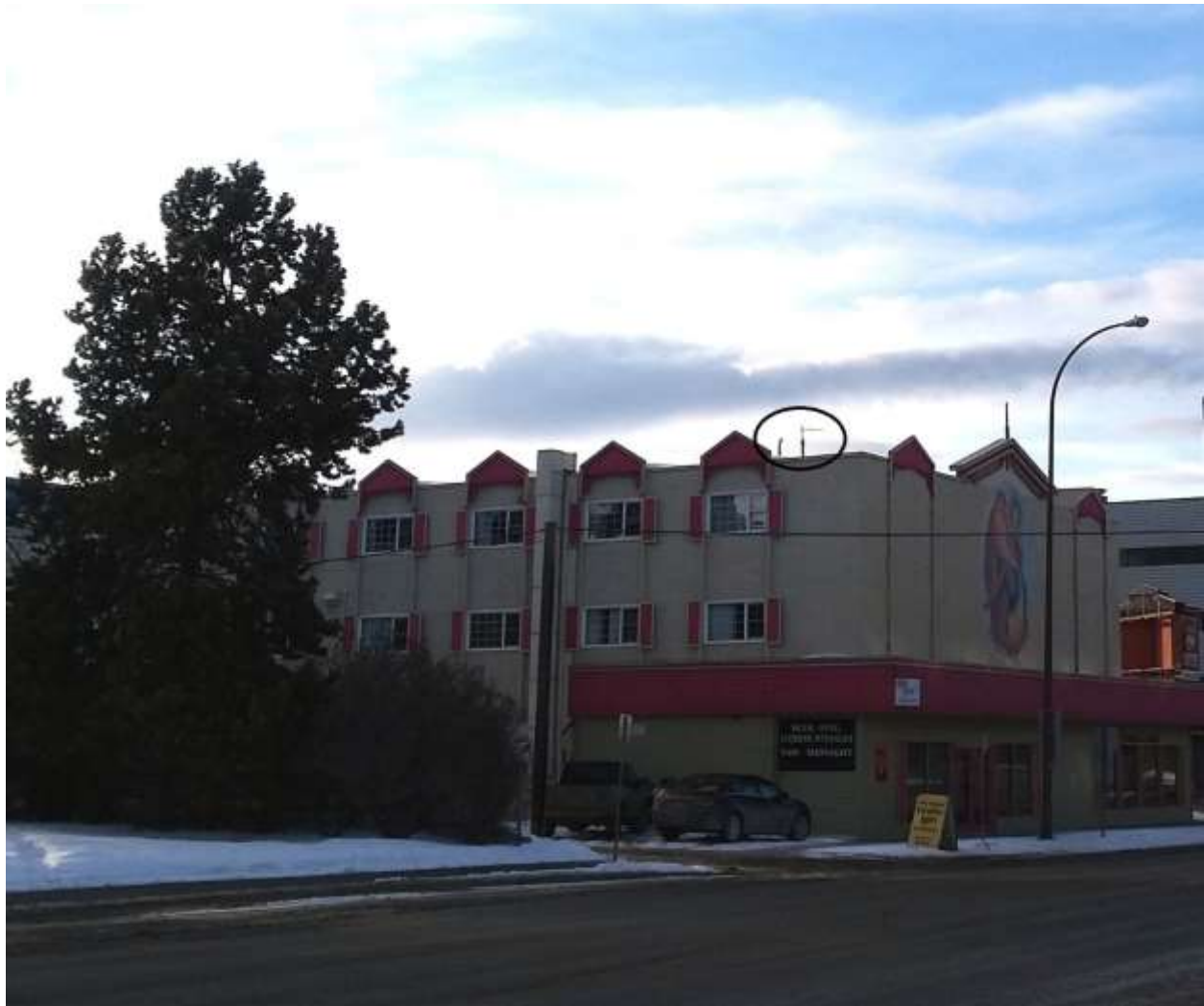
Figure 5 - Base GNSS Antenna Installation
