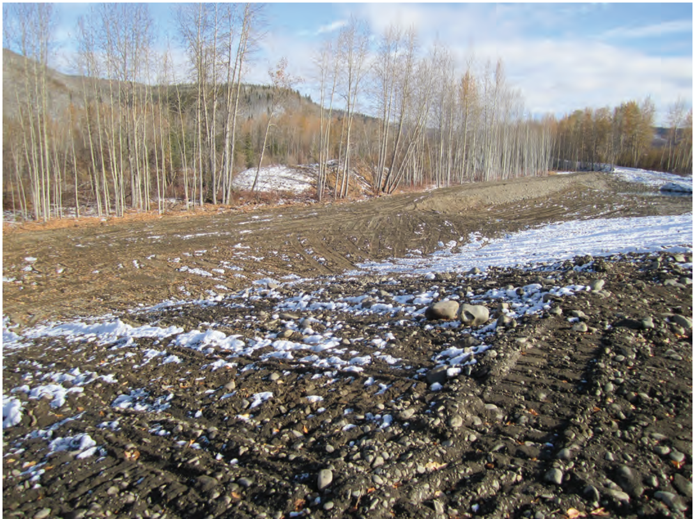
Figure 3. Berm/trail created to alleviate flooding.
