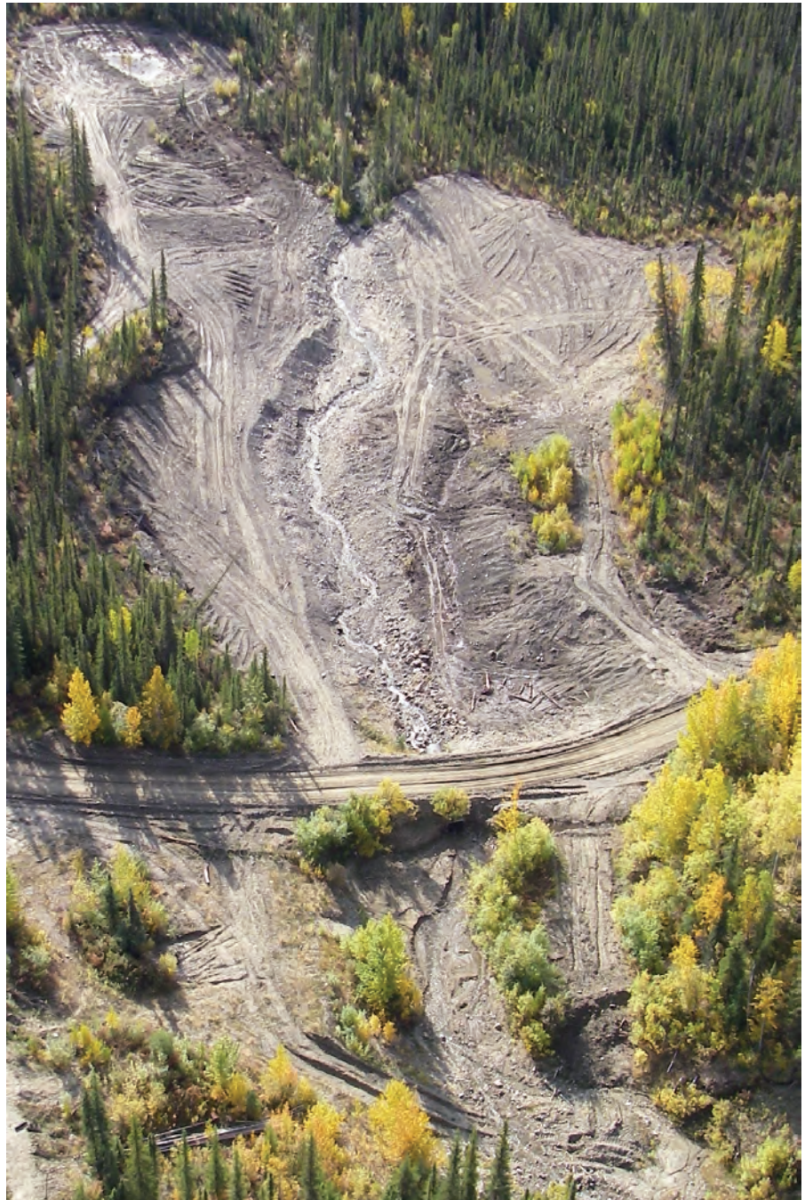
Figure 2. Sloped, contoured and scarified area along Haggart Creek Road, near Mayo. Reclaimed area was covered in fines to enhance re-vegetation.
