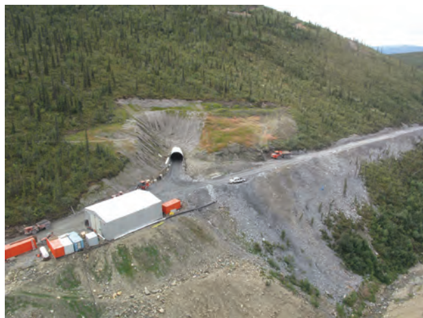
Figure 8. Portal at Bellekeno Mine.
