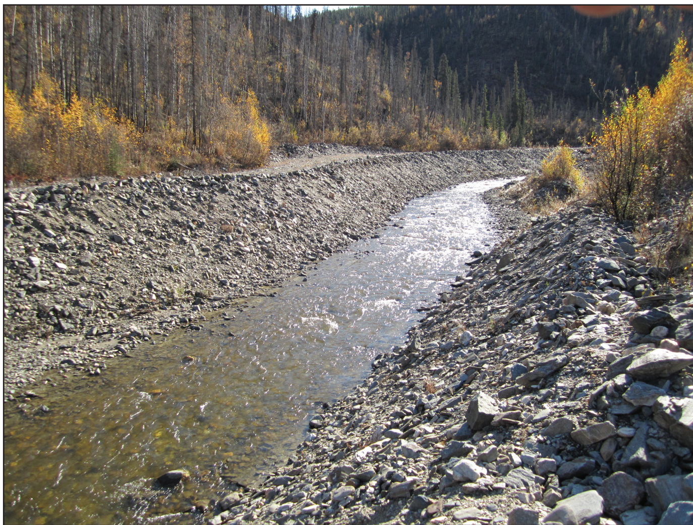
Figure 2. Stabilized creek channel.
