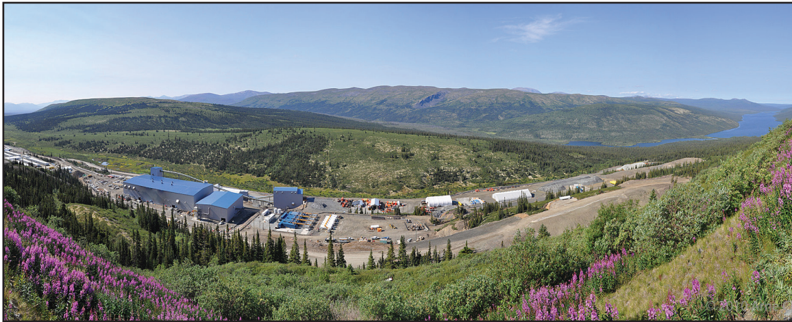
Figure 1. Yukon Zinc's Wolverine mine site, July 2010.
