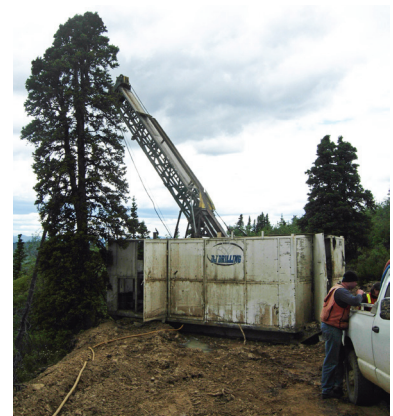
Figure 26. Drilling the Flex Zone at the Charlotte property of Ansell Capital Corp.
