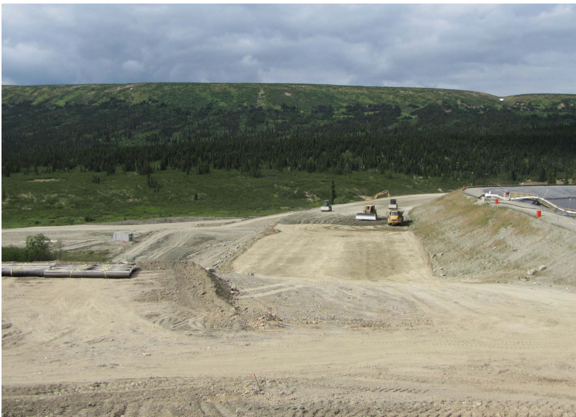
Figure 3. Equipment placing and compacting material on the tailings dam lift. Photo - courtesy of Glenn Ford, Water Resources.
